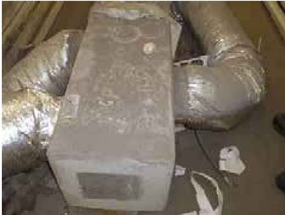
Photo 5: Typical nonACM white HVAC duct mastic sampled during this inspection.
