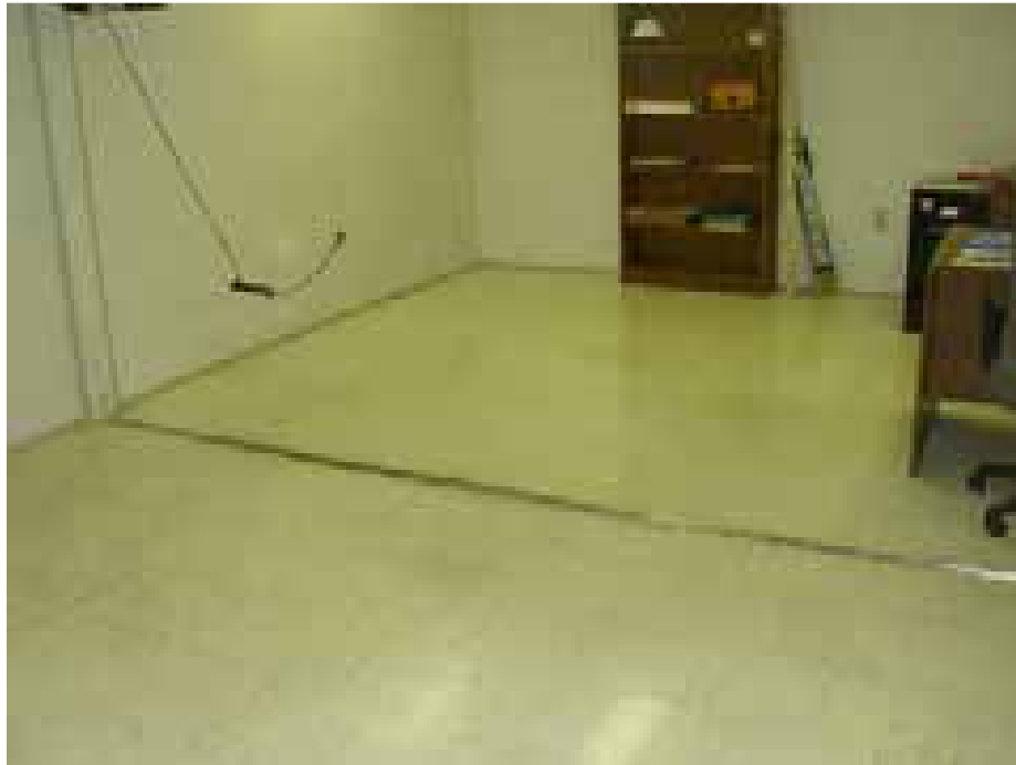
Photo 15: NonACM white 12"x12" VFT sampled during this inspection.
