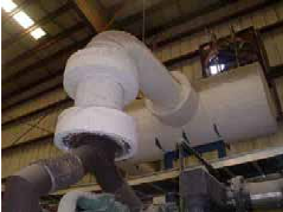
Photo 10: NonACM white generator muffler exhaust insulation sampled during this inspection.
