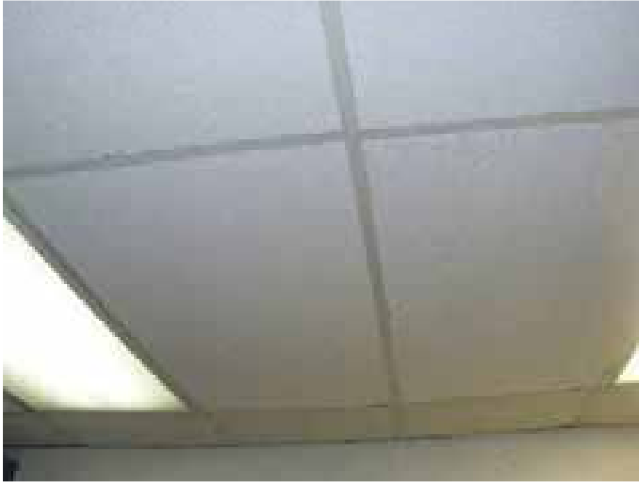
Photo 3: Typical nonACM 2'x4' ceiling tile sampled during this inspection.
