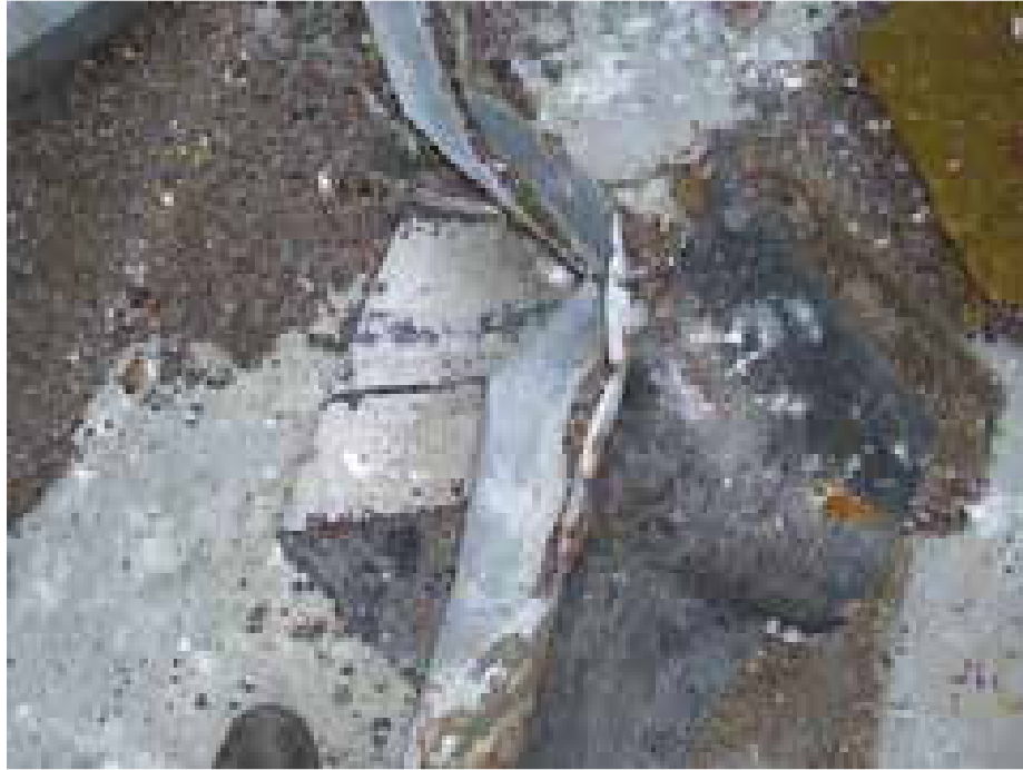
Photo 19: NonACM roof edge flashing sampled at the Ash building during this inspection.
