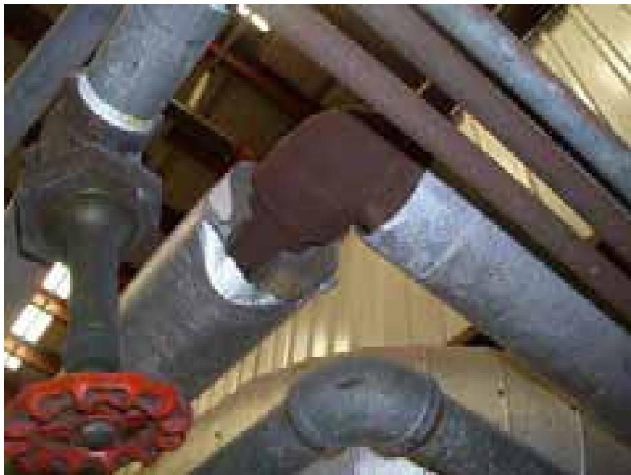
Photo 8: Typical nonACM pipe insulation sampled during this inspection.
