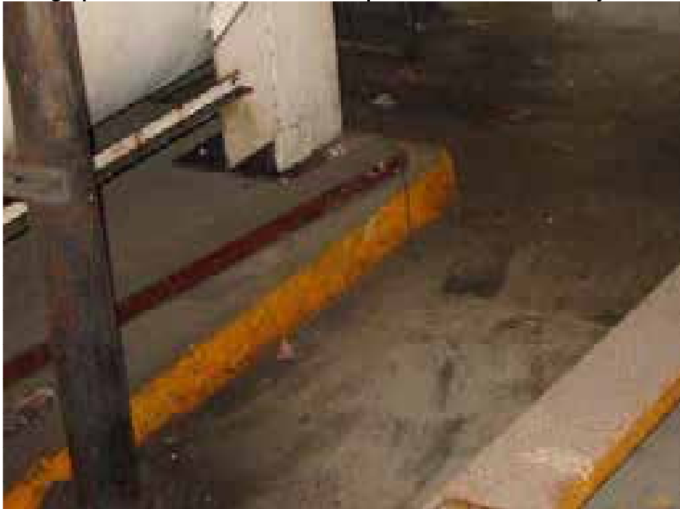
Photograph #4: Concrete floor curbing in Resource Recovery Building
