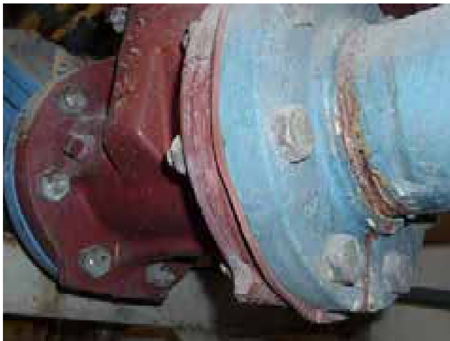
Photo 12: NonACM red gasket sampled during this inspection.
