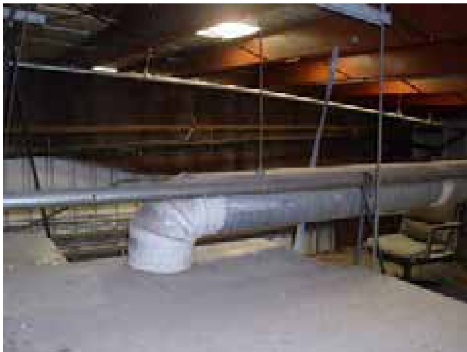
Photo 6: NonACM white metal pipe mastic sampled during this inspection.
