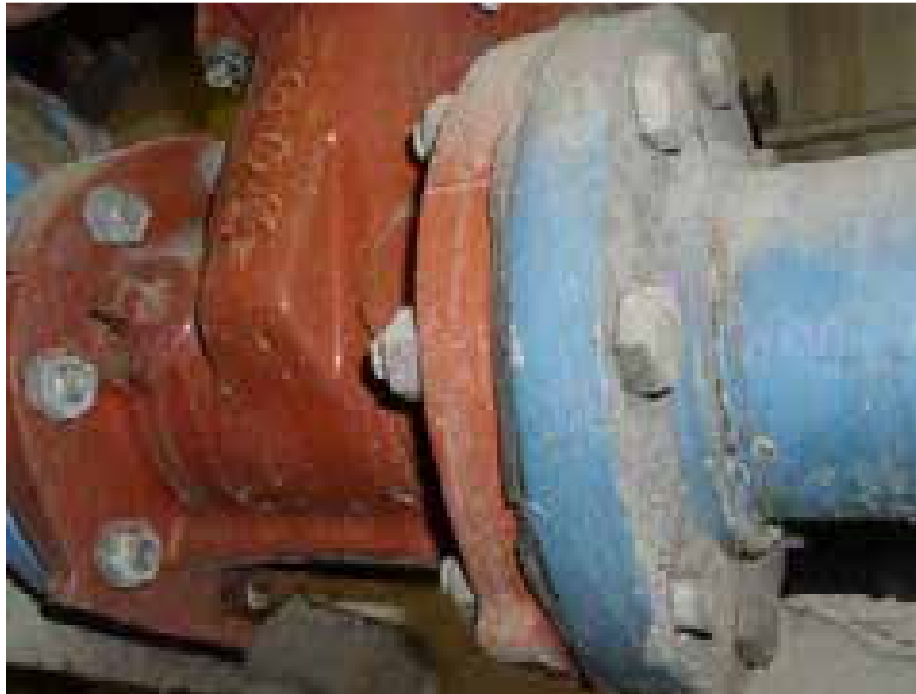
Photo 11: NonACM black gasket sampled during this inspection.
