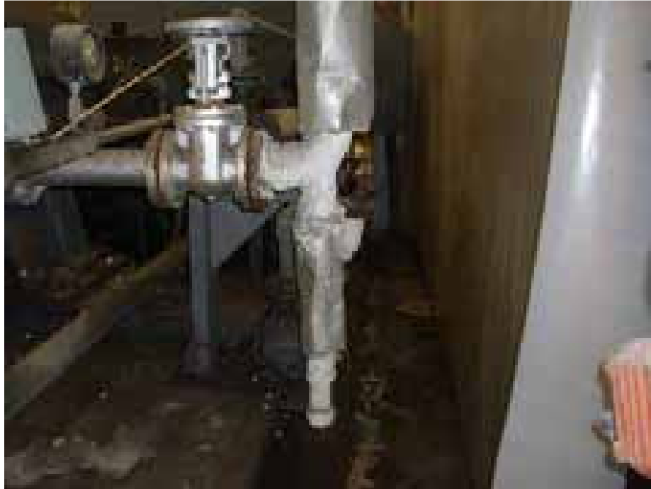
Photo 13: Typical nonACM pipe insulation sampled during this inspection.
