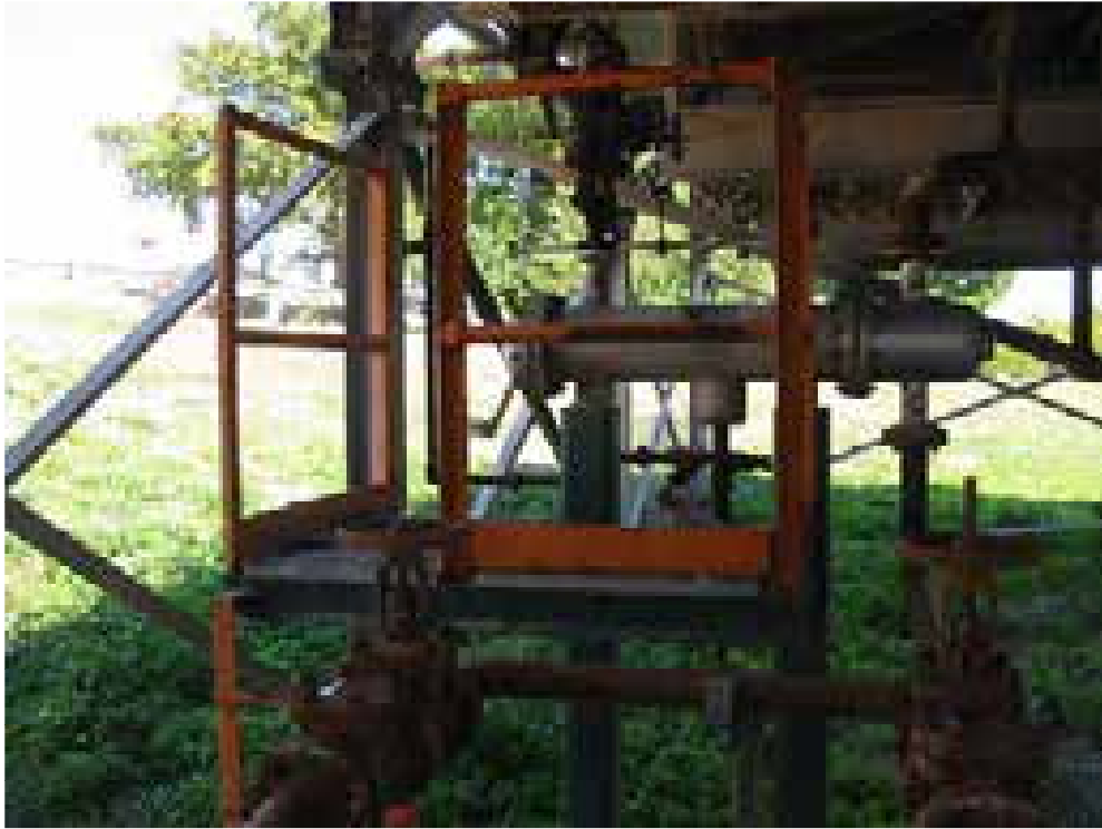
Photograph #13: Safety railings and ladder under Raised Cooling Tower Structure.
