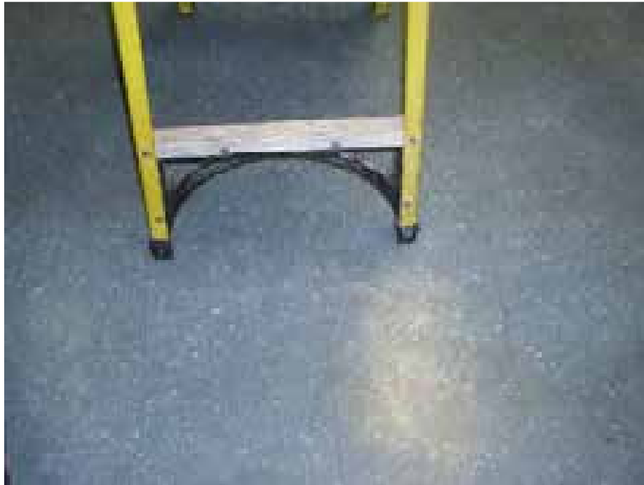
Photo 7: Typical nonACM 12"x12" blue VFT with glue sampled during this inspection.
