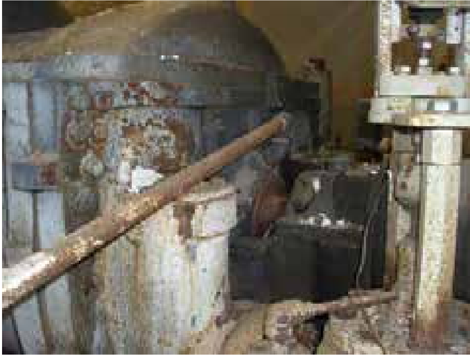
Photo 9: Typical nonACM white pipe insulation debris sampled during this inspection.
