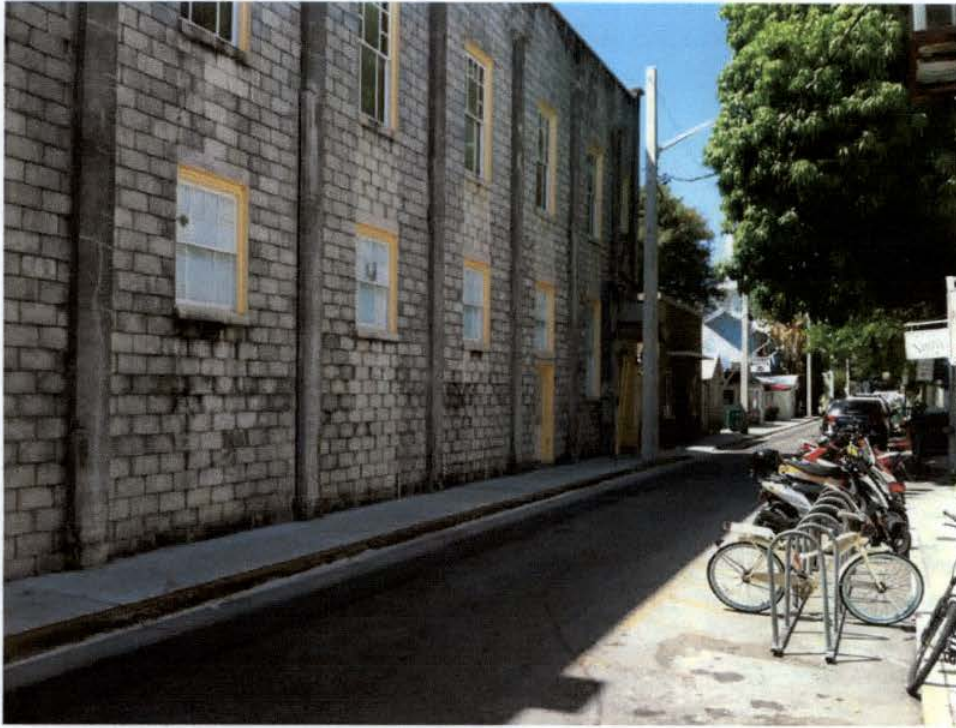
VIEW DOWN APPELROUTH LANE FROM DUVAL STREET
