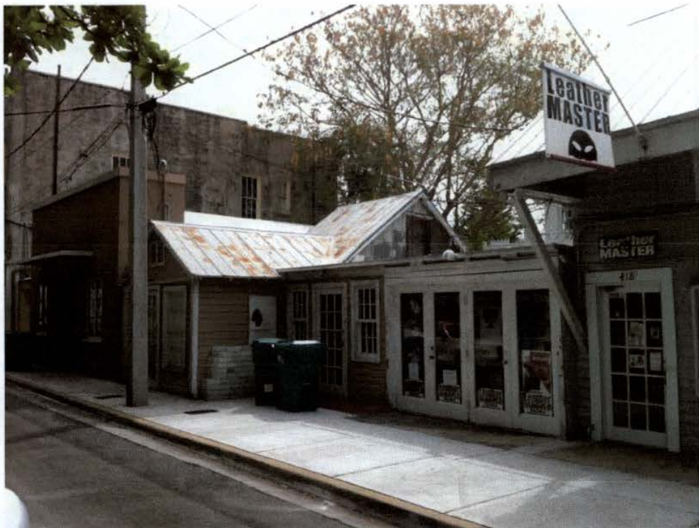
418-420 APPELROUTH LANE - AREA OF ROOF REPLACEMENT
