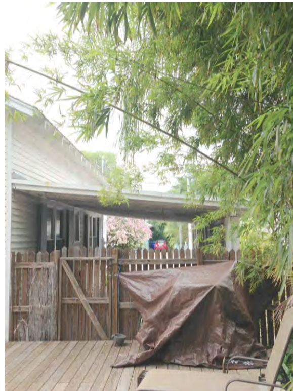
FIGURE 4 REAR VIEW OF CAR PORT
