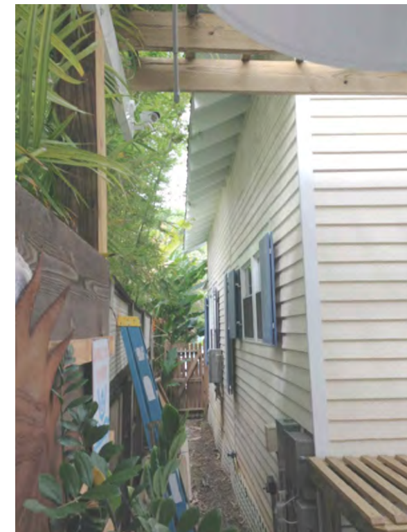
FIGURE 6 REAR RIGHT VIEW OF HOUSE
