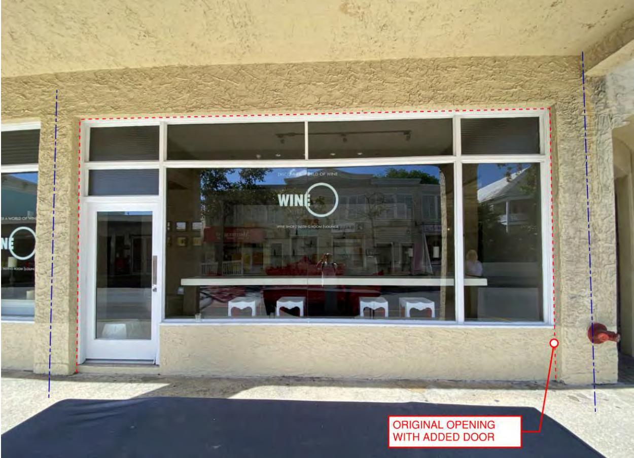
Bay 7 – existing conditions
