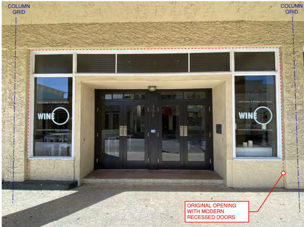
Bay 6 – existing conditions
