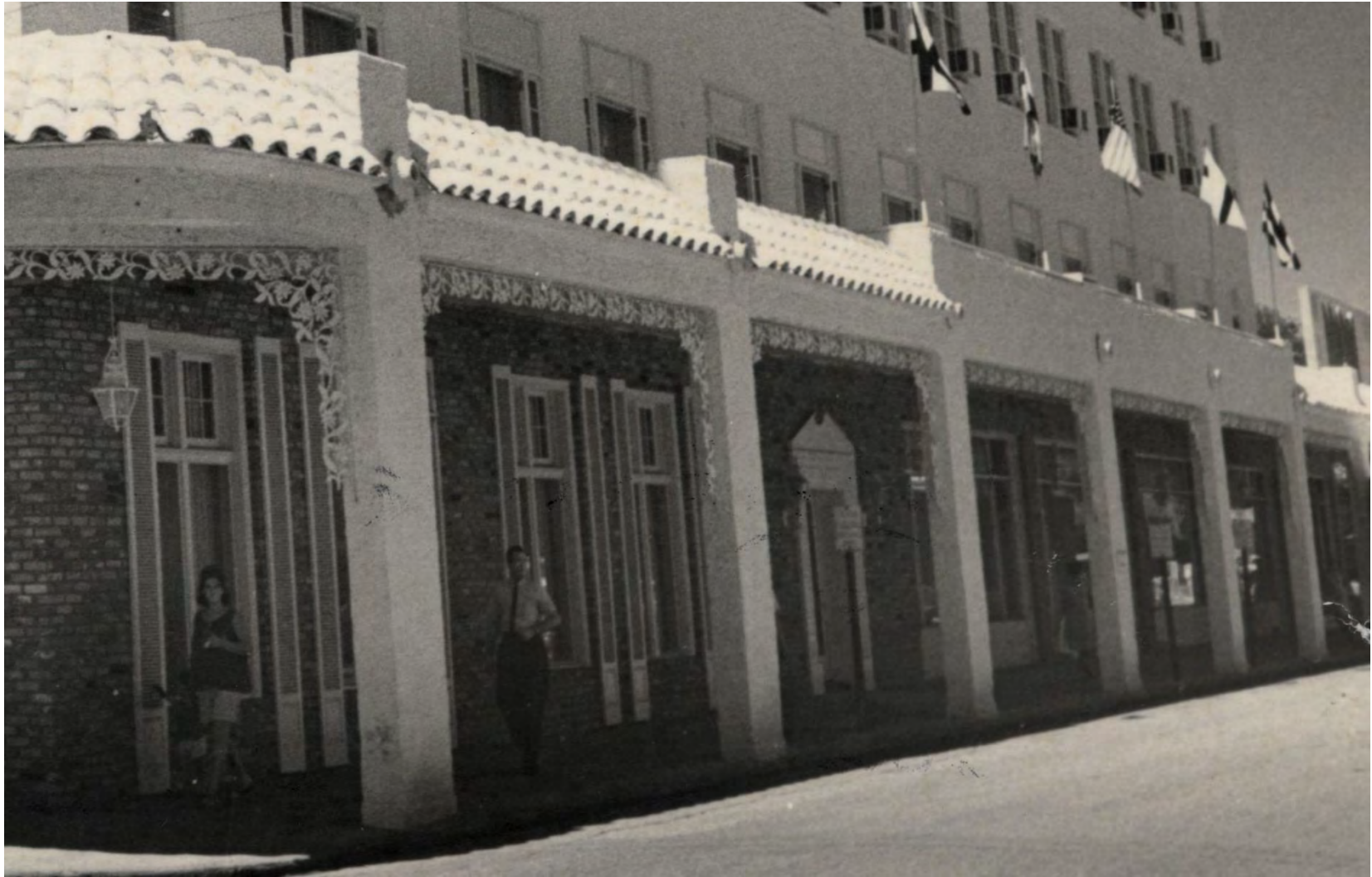
Detail of 1962 photograph. Monroe County Library.
