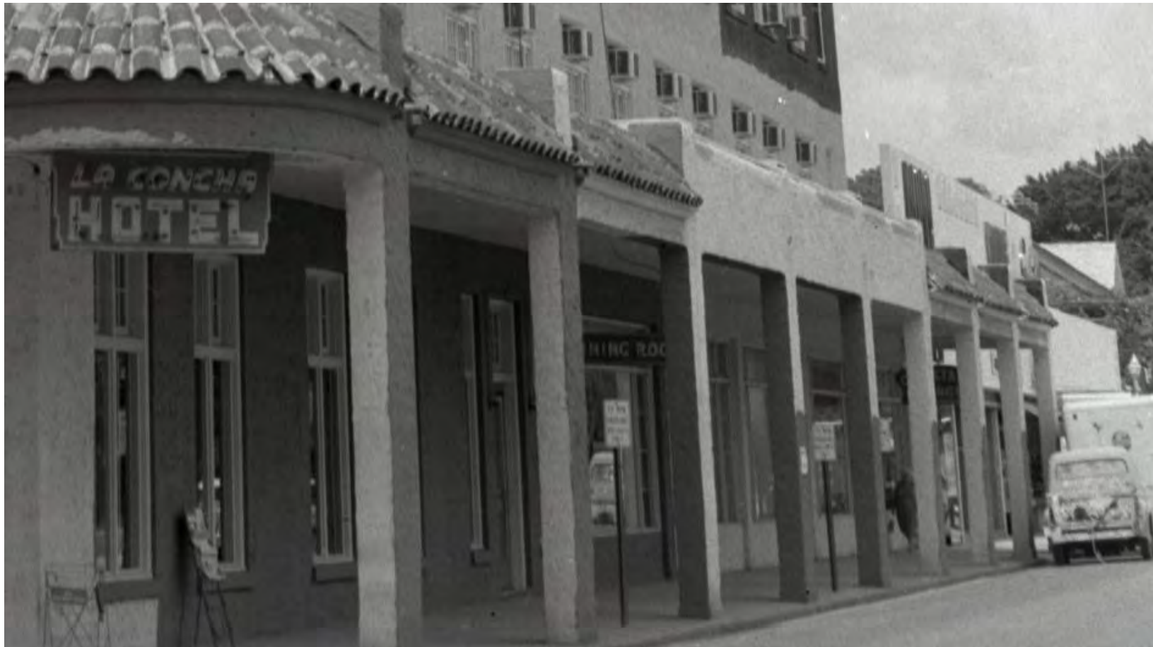
Detail of 1957 photograph. Monroe County Library.
