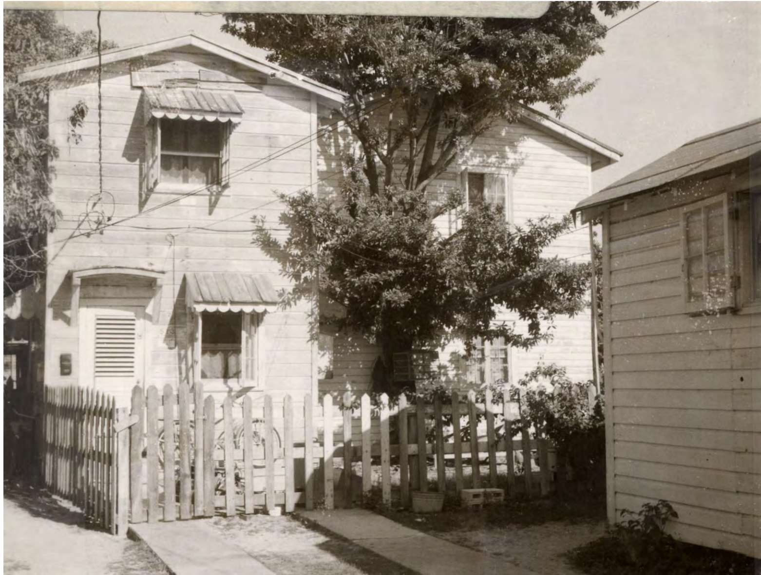
Building under review, historically known as 513 Catherine Street, circa 1965. Monroe County Library.
