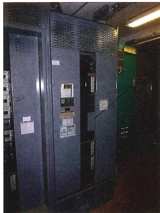
2000A 277/480V PANEL MAIN ELECTRICAL ROOM
