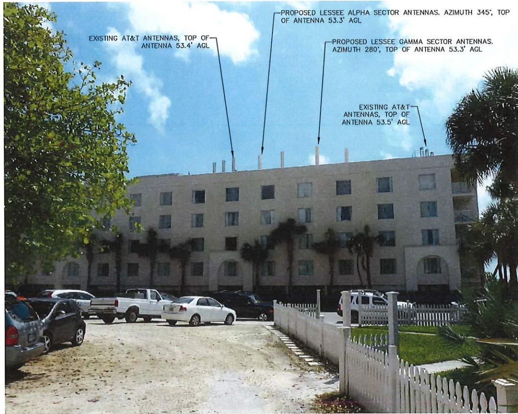
NORTHWEST BUILDING ELEVATION
