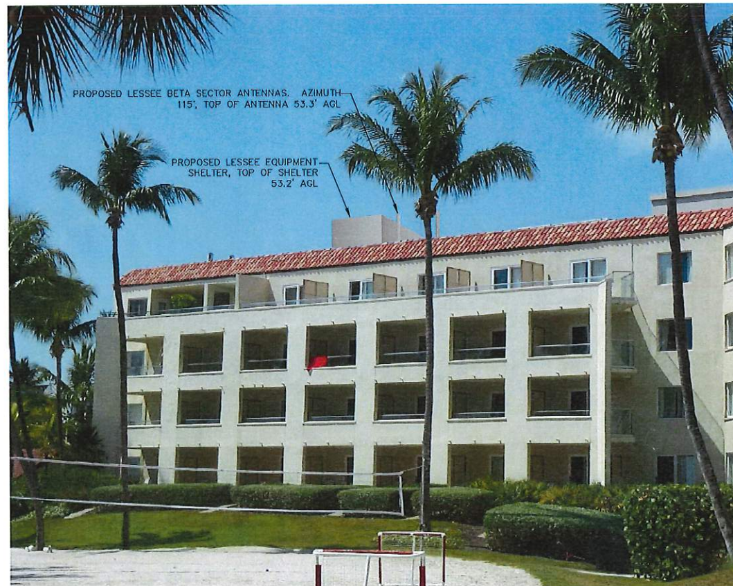
SOUTHEAST BUILDING ELEVATION
