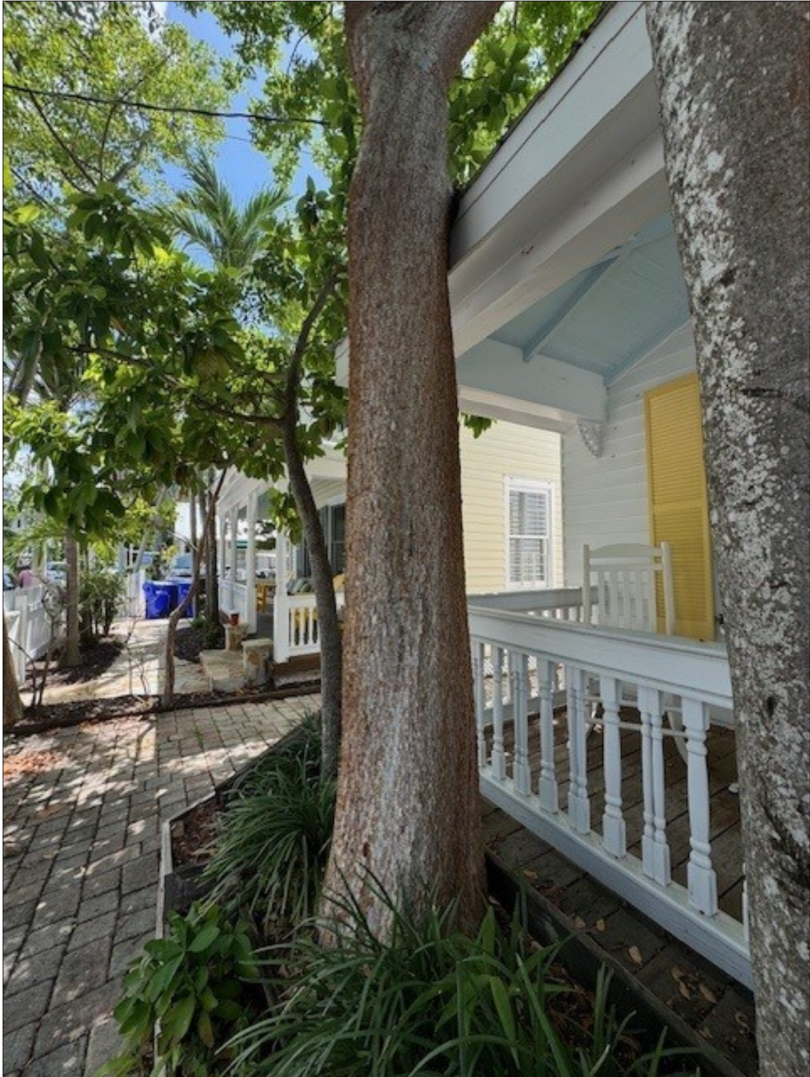
The lower trunk is encroaching upon the front porch.
