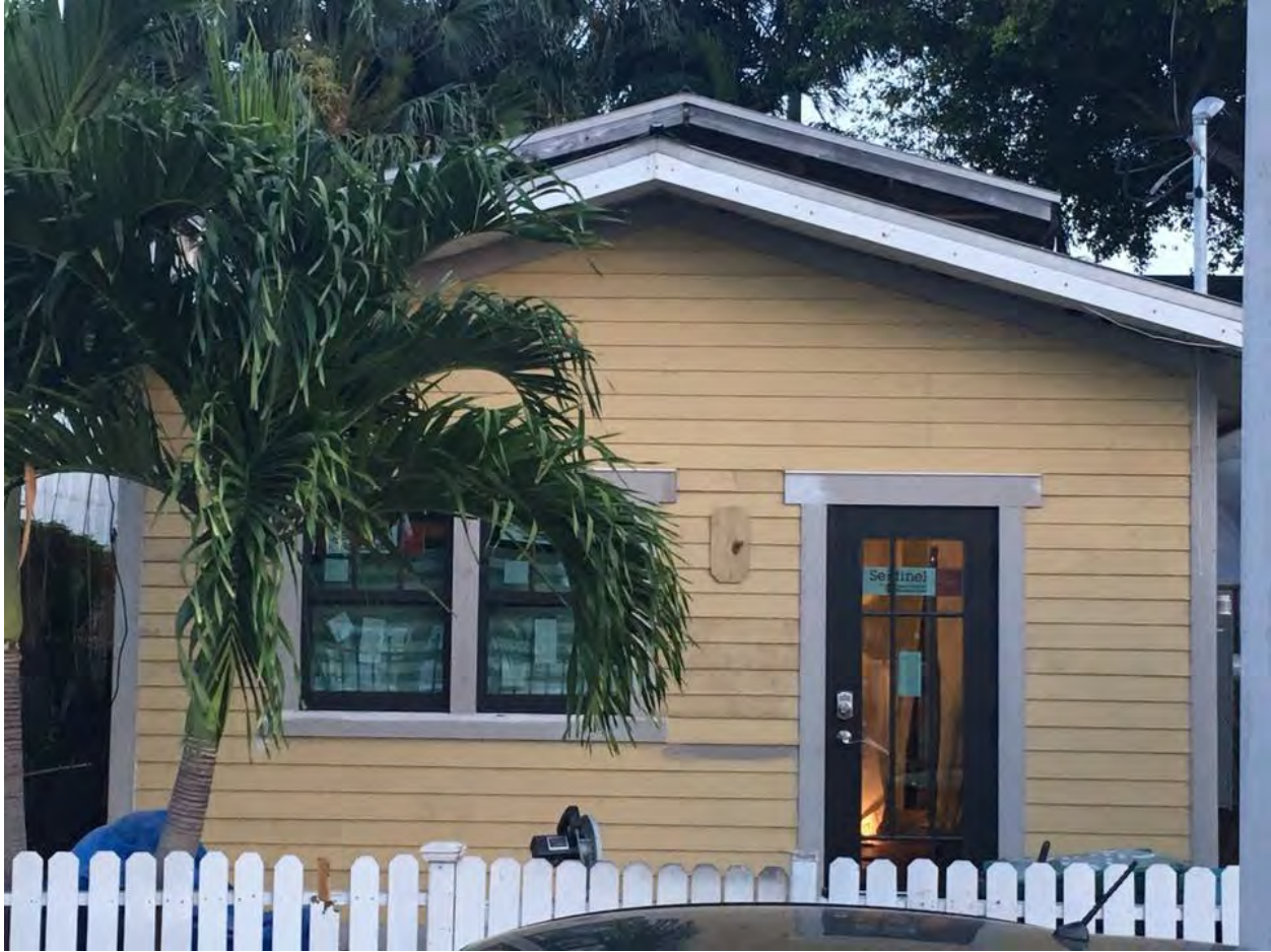
904 Olivia front elevation (in progress renovation)
