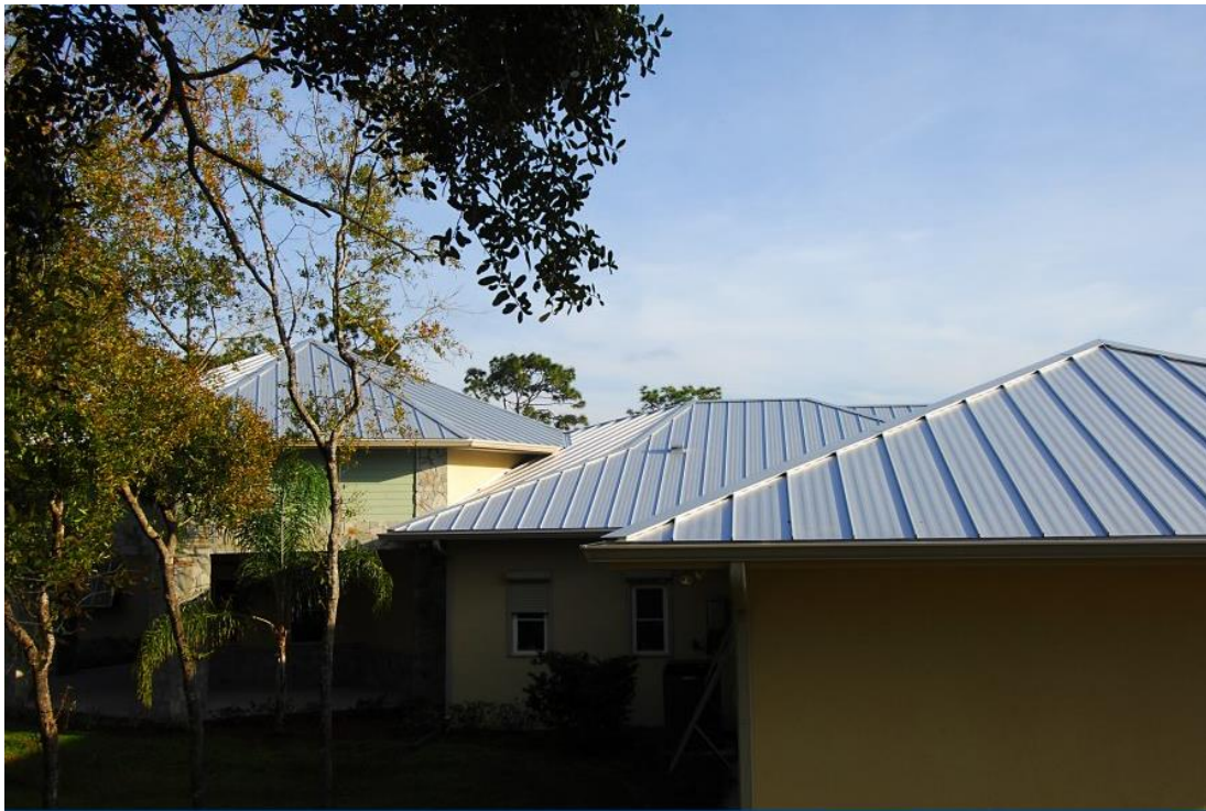
Examples of 1-inch standing seam roof
