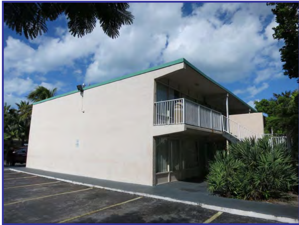
Southeast side of Building C
