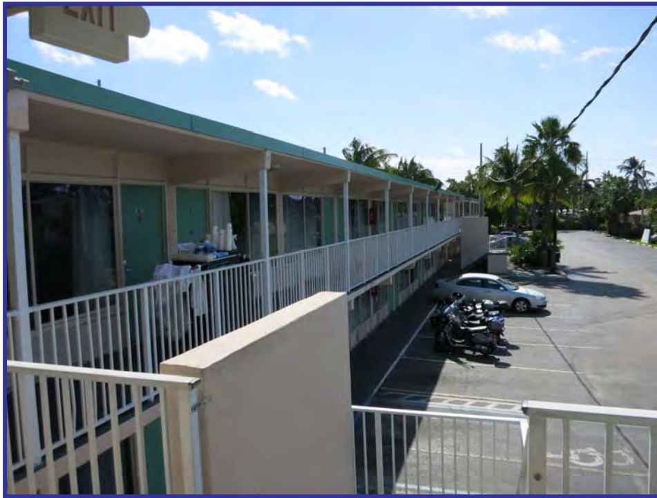
The north elevation of building A - view from the second floor
