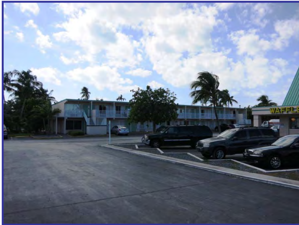
View of the subject as seen from North Roosevelt Boulevard
