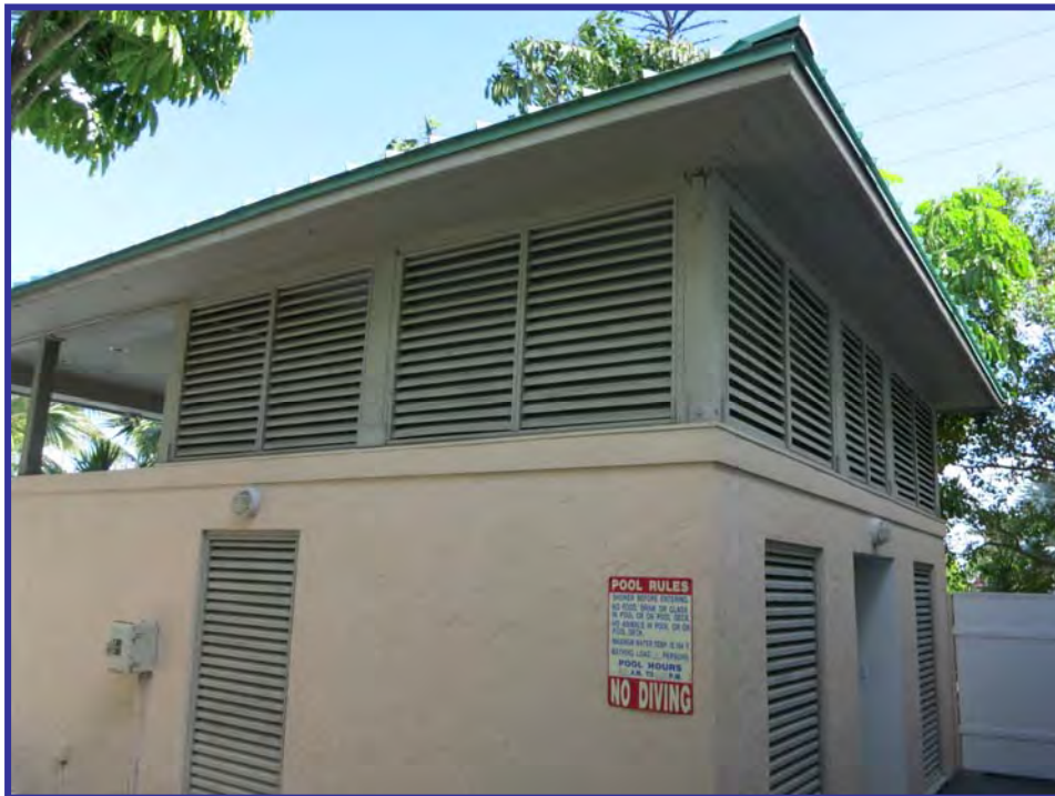
Pool cabana - showers and bathroom
