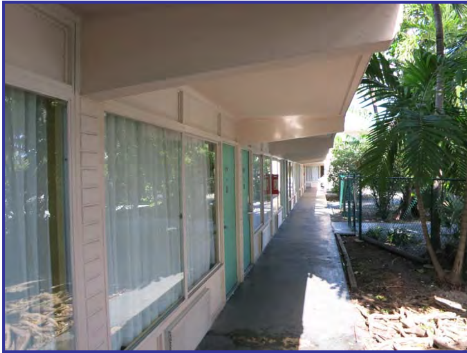
View looking north along the east elevation of building B
