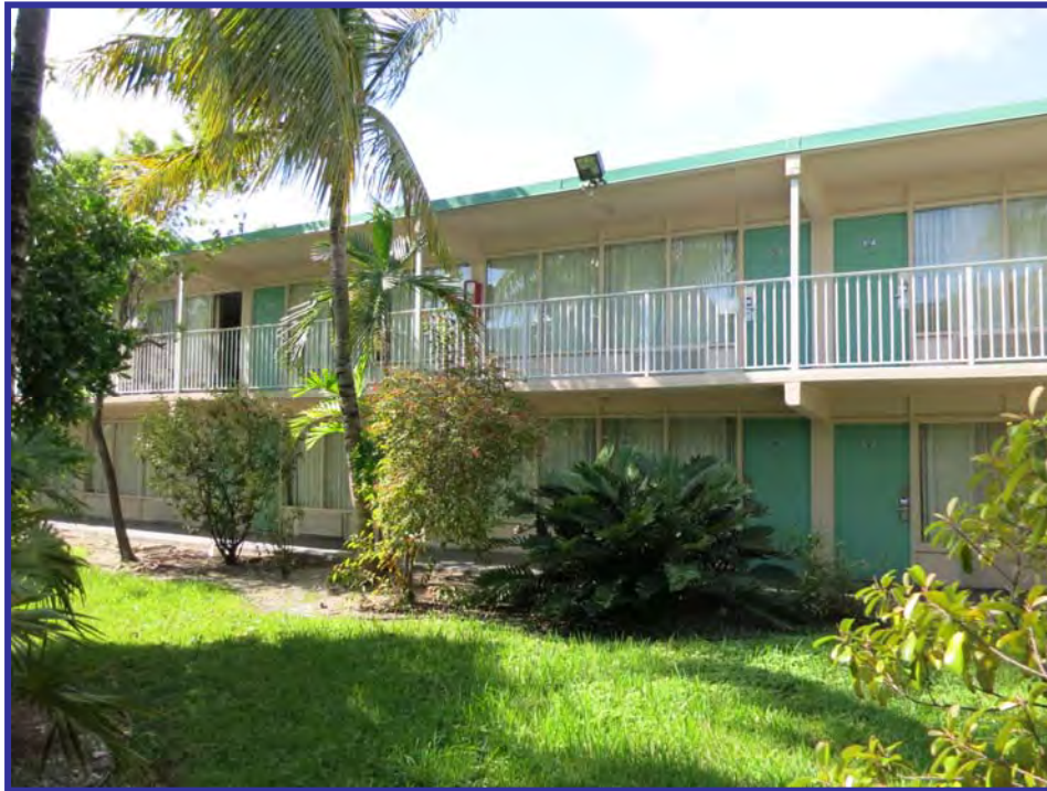
Building B as seen from the pool area
