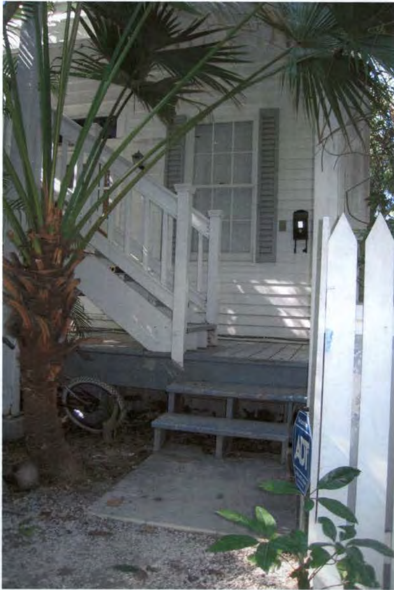
BOTTOM OF REAR STAIRS
