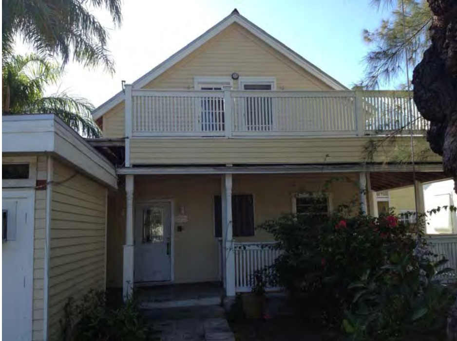
Current street side view of the structure
