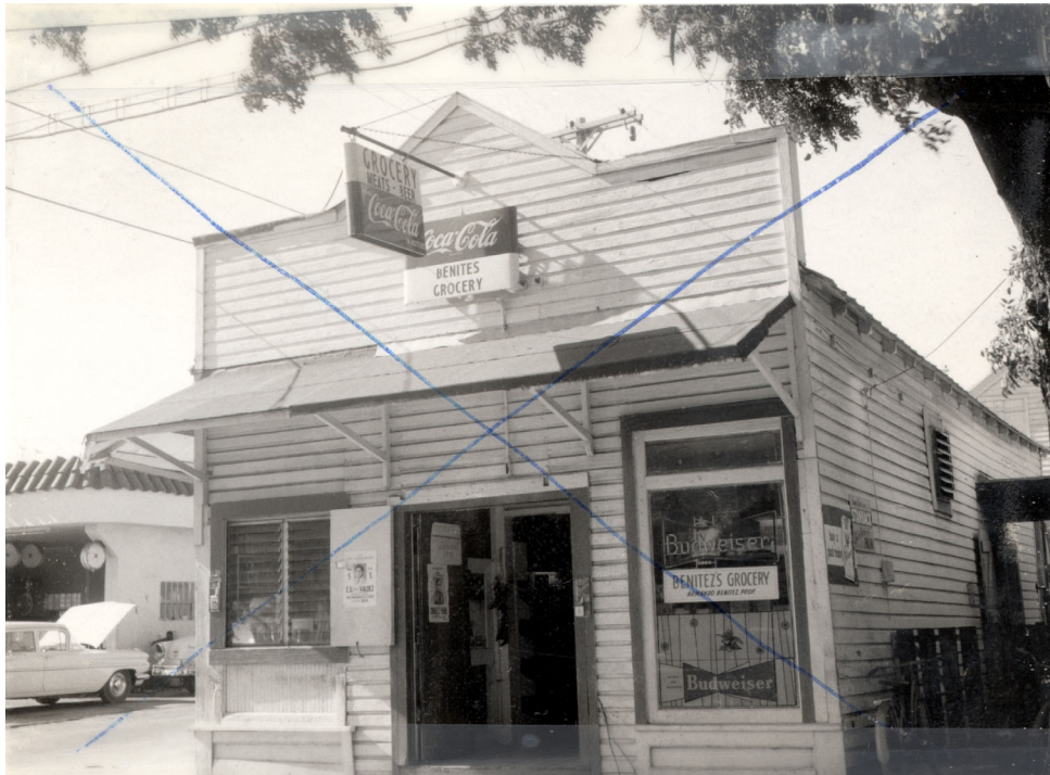
728 SIMONTON ST. | 1965 Monroe County Property Appraiser. Note: Included as an example of neighborhood grocery store, with storefront windows, and centralized entrance doors.
