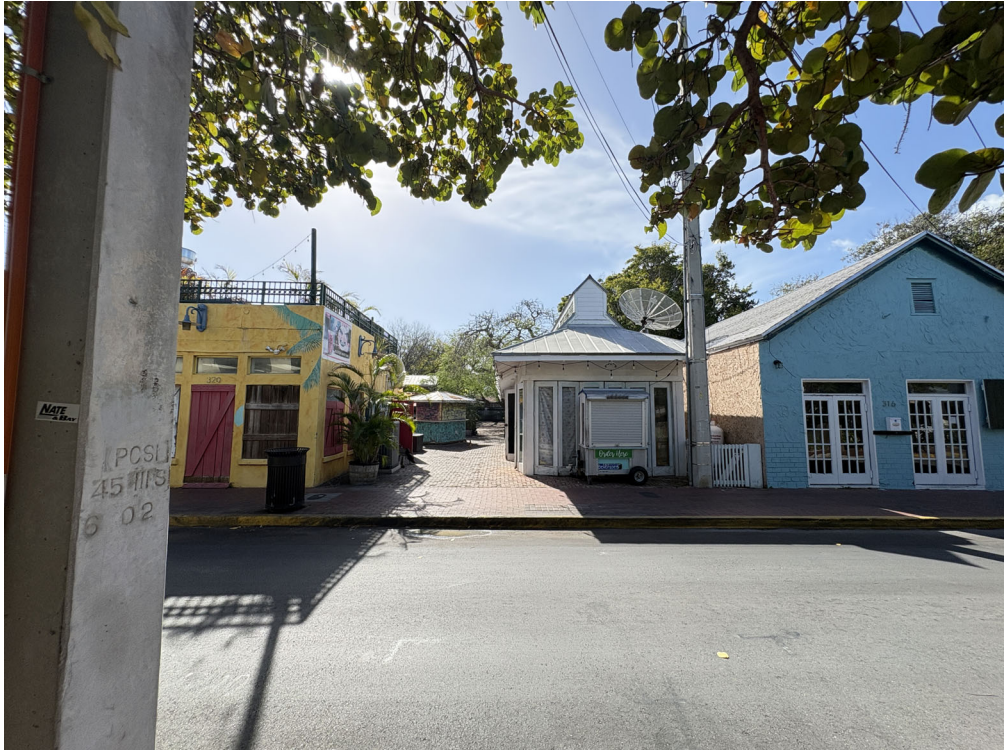
324 PETRONIA ST. | North elevation [2026.03.10].
