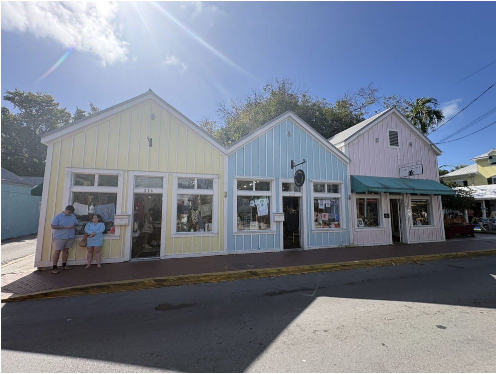
314 PETRONIA ST. | North elevation [2026.03.10].
