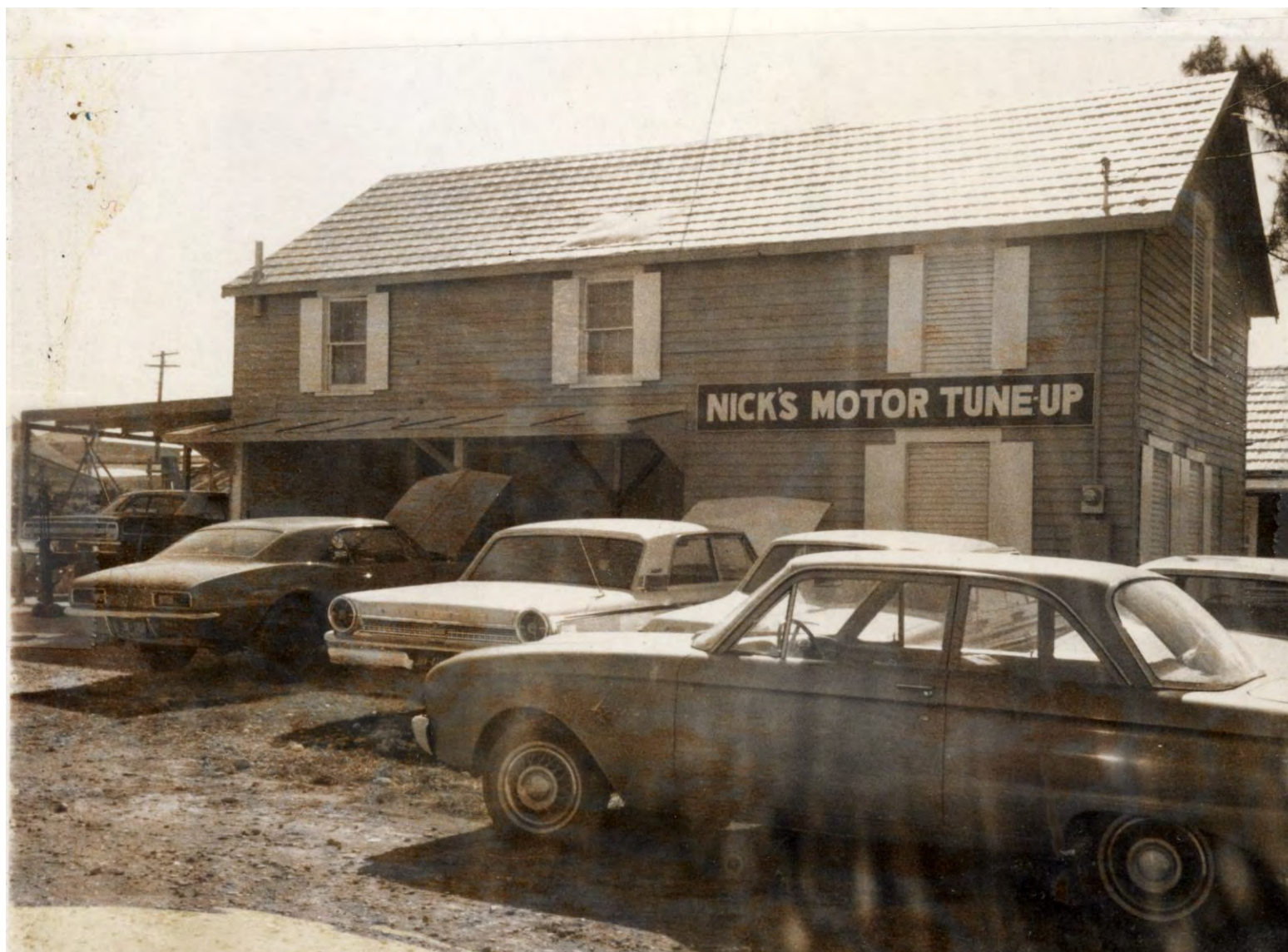
Structure on site circa 1965. Monroe County Library.
