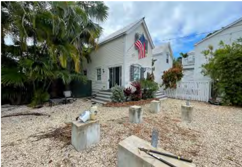
Site with accessory structure.
