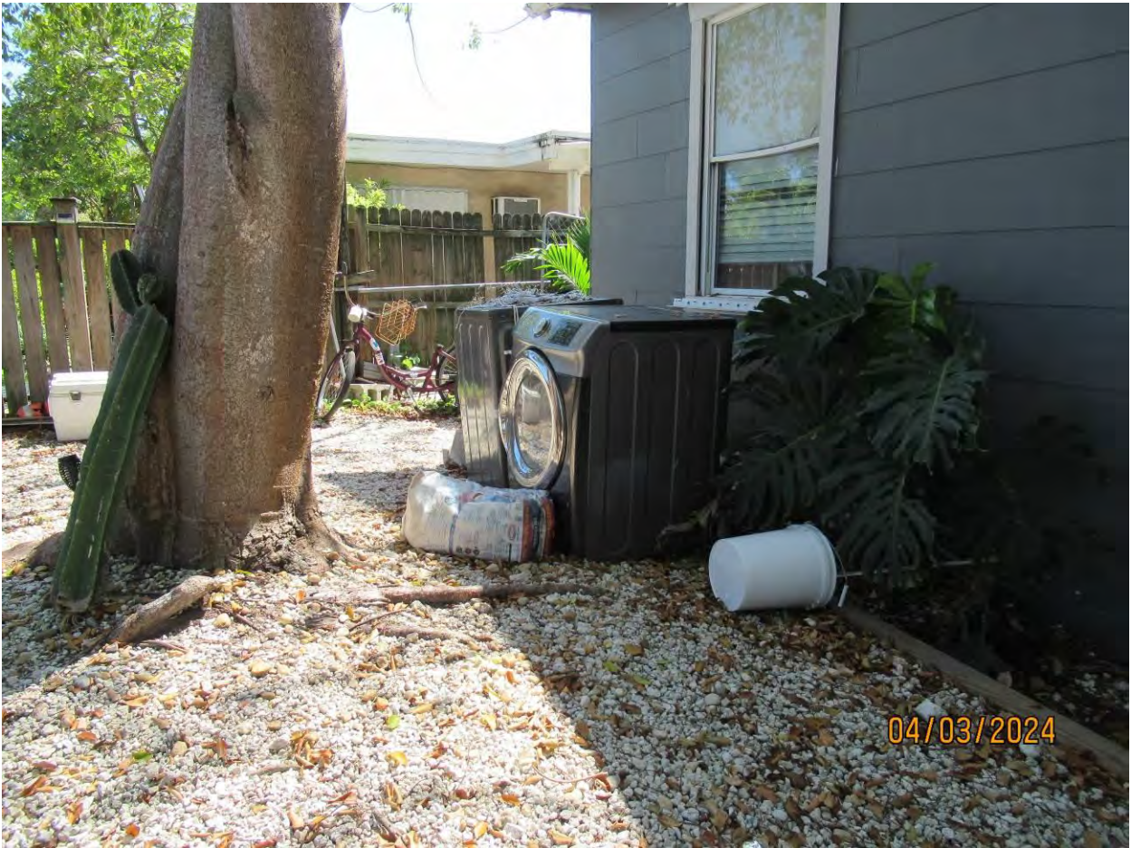
Photo of base of tree in relation to structure.
