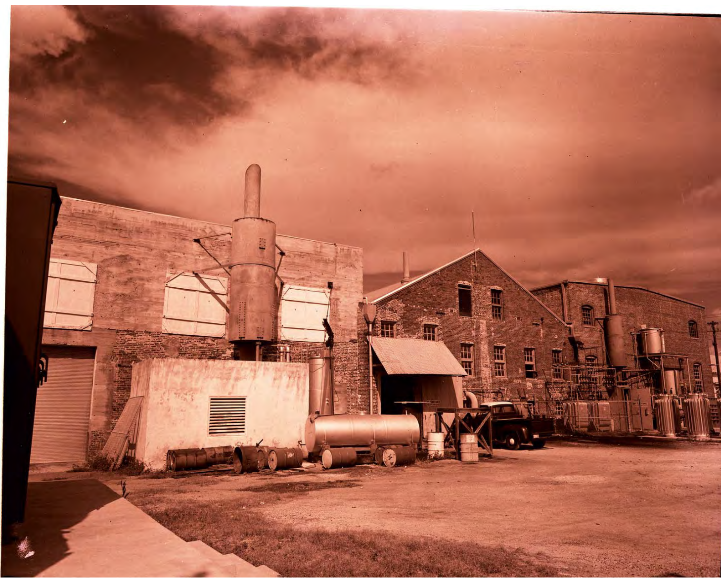
The old city electric plant and substation. Wright Langley Collection. Monroe County Library.
