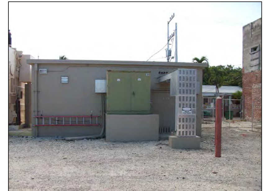
BUILDING TO BE DEMOLISHED
