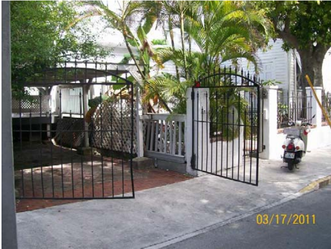
Above – unlocked gates for off-street parking space Below – left side porch
