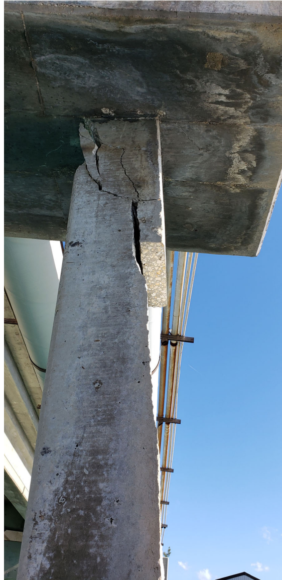
Figures 2 and 3. Bottom of the pier snapped and heavy damage to the top.
