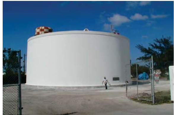
700,000 Gallon Concrete Water Tank
