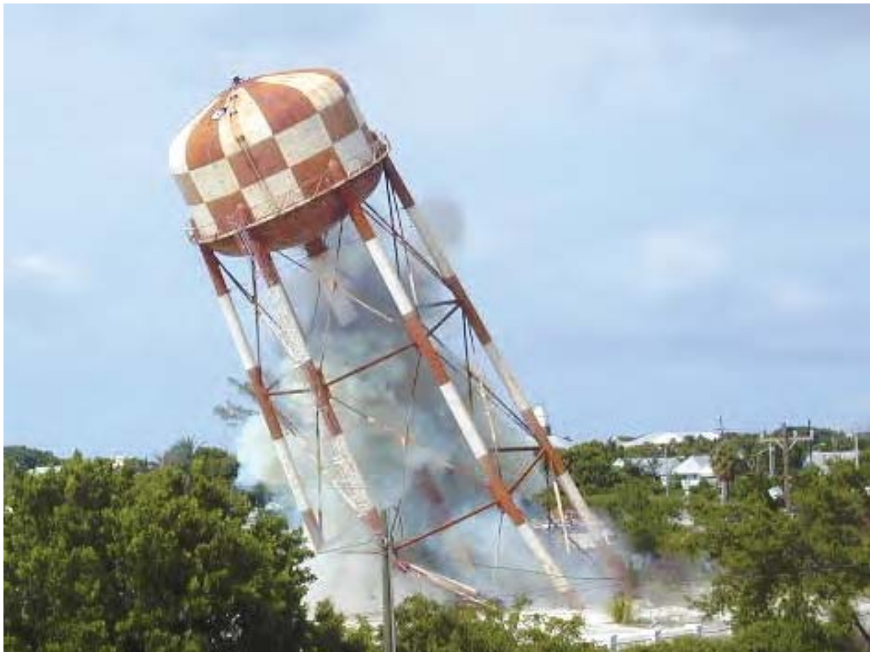
Water Tank Demolition, NAS Key West
