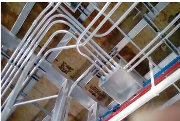
Marathon Utility & Maintenance Building
