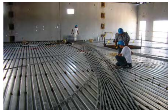
Slab Rough-In, Marathon High School
