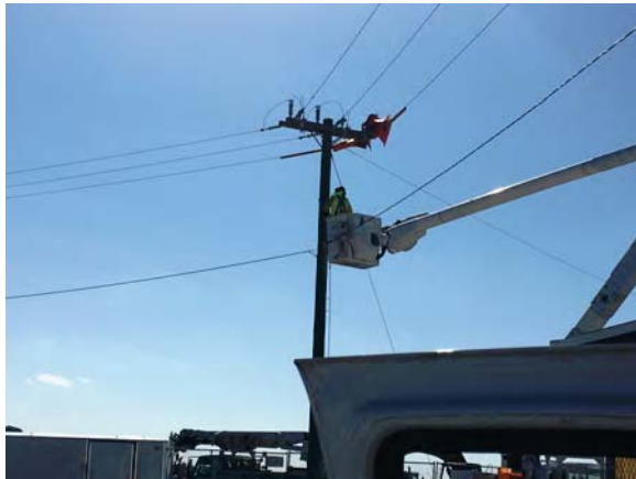
Installing Guy Wire NAS KW
