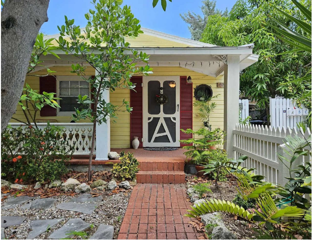
Photo showing 737 Elizabeth Street which currently has red shutters.
