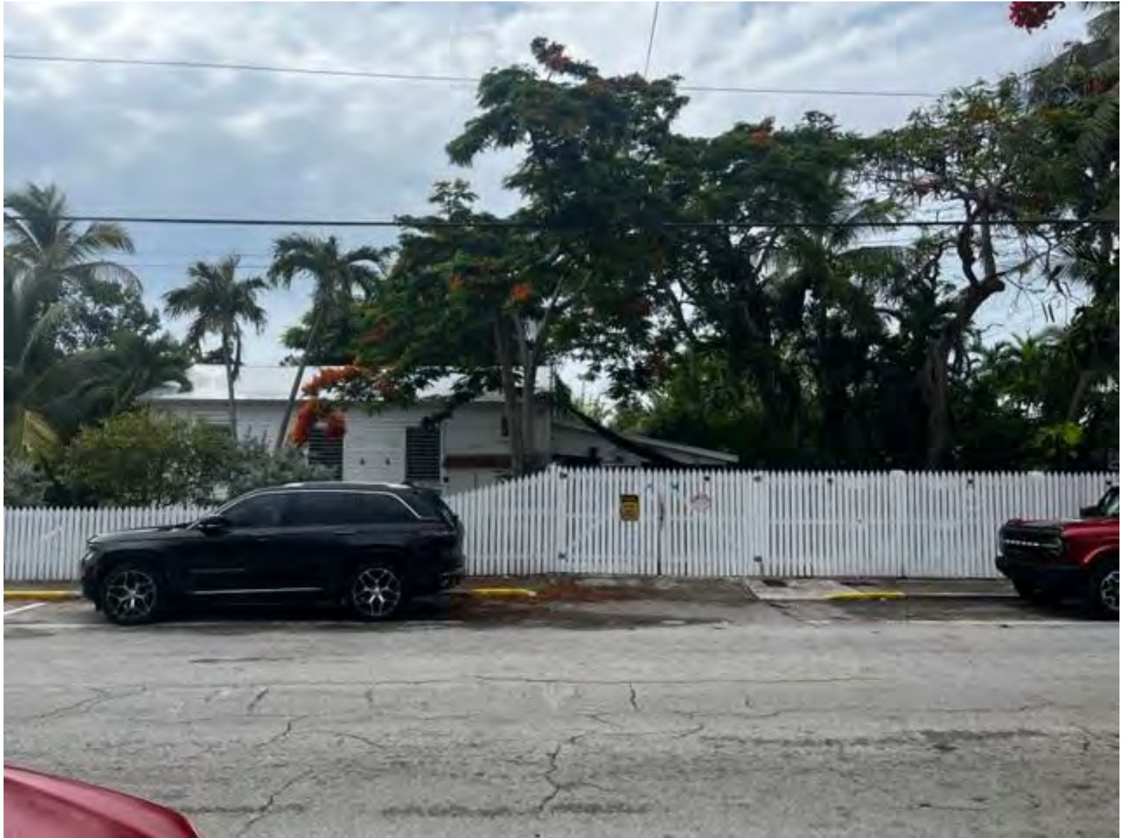
North elevation facing Catherine Street.
