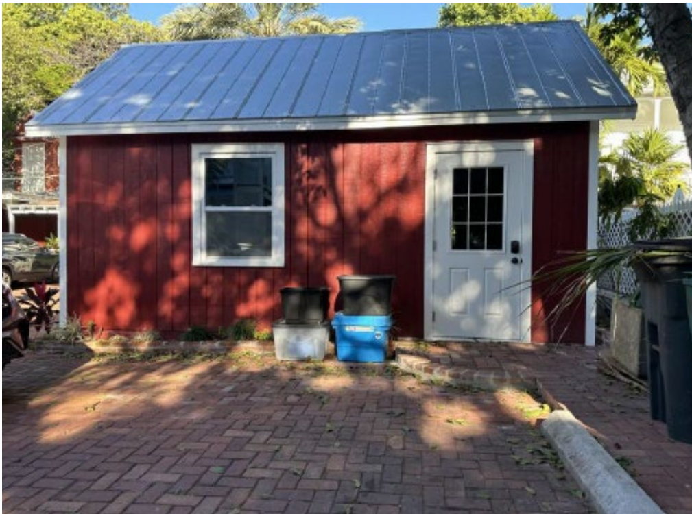
Photo of shed under review (entry elevation).
