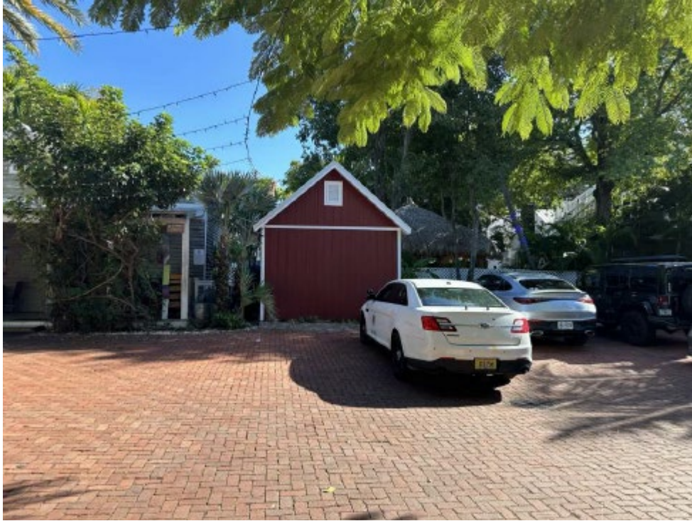
Photo of shed under review from rear parking lot.
