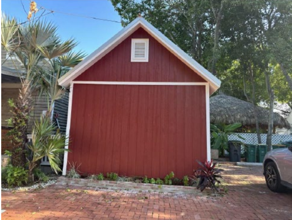
Photo of shed under review (side elevation).
