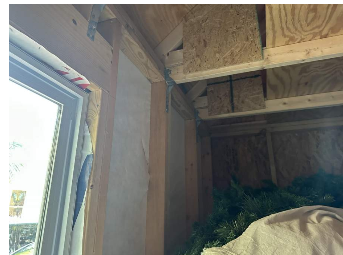
ROOF TRUSSES TO WALL CONNECTION
