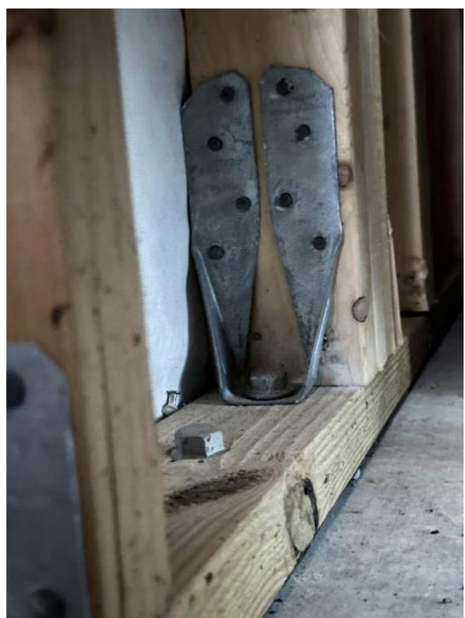
WALL PLATE AND WALL STUD CONNECTION
