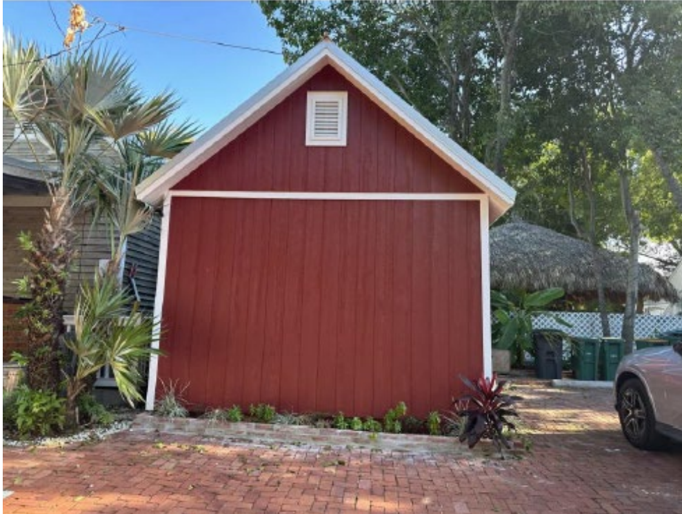
Photo of shed under review (side elevation).
