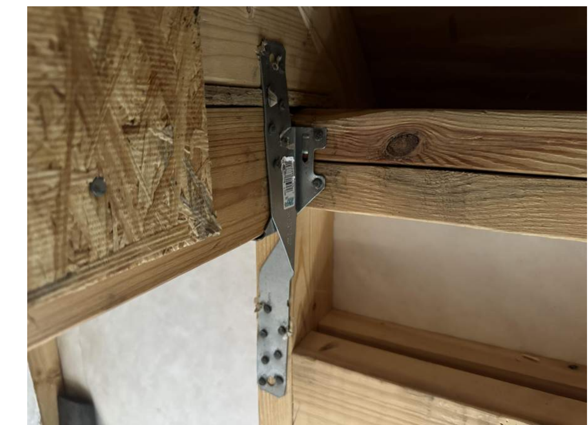
ROOF TRUSSES TO WALL CONNECTION
