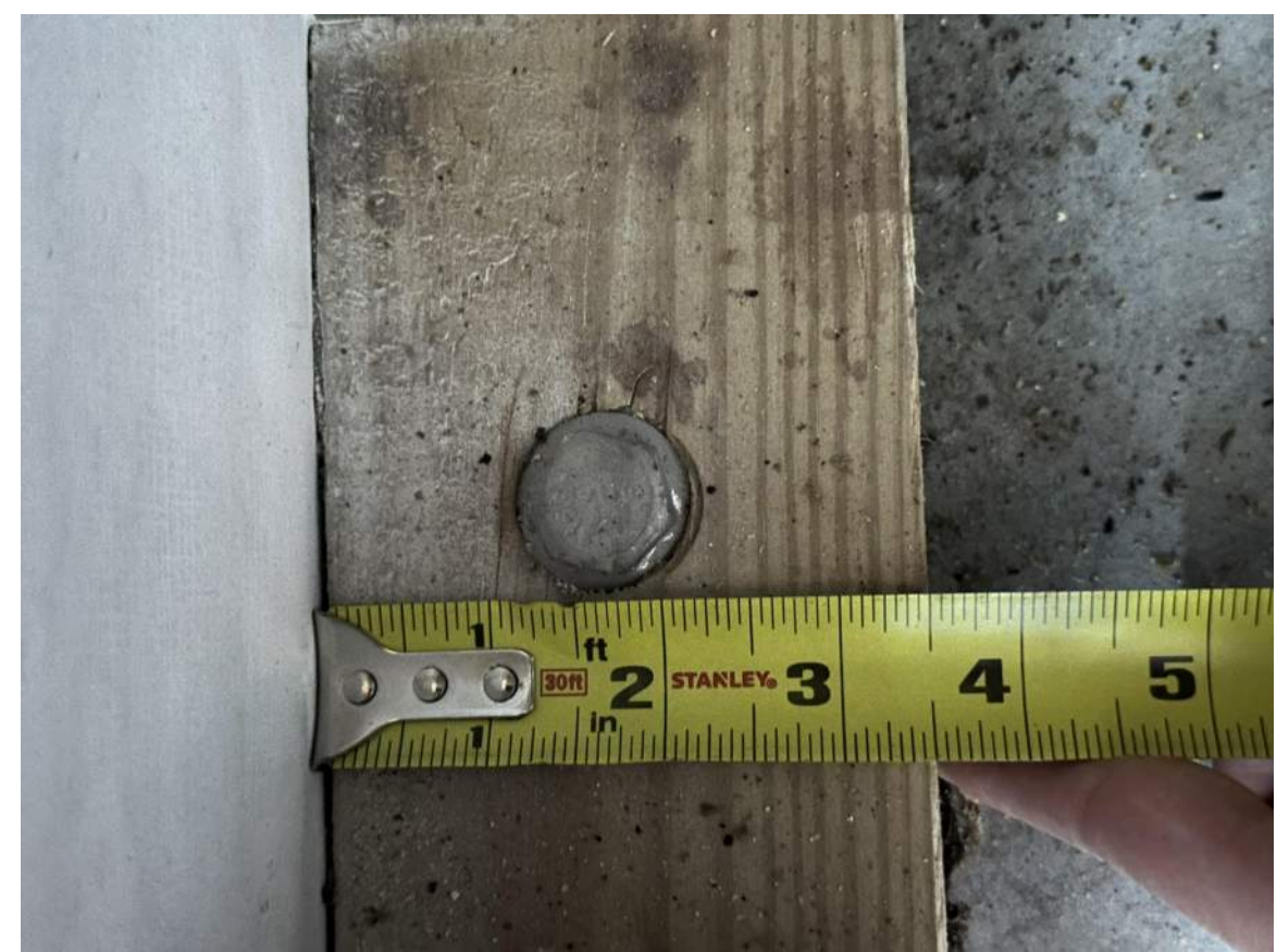
WALL PLATE AND SLAB CONNECTION
