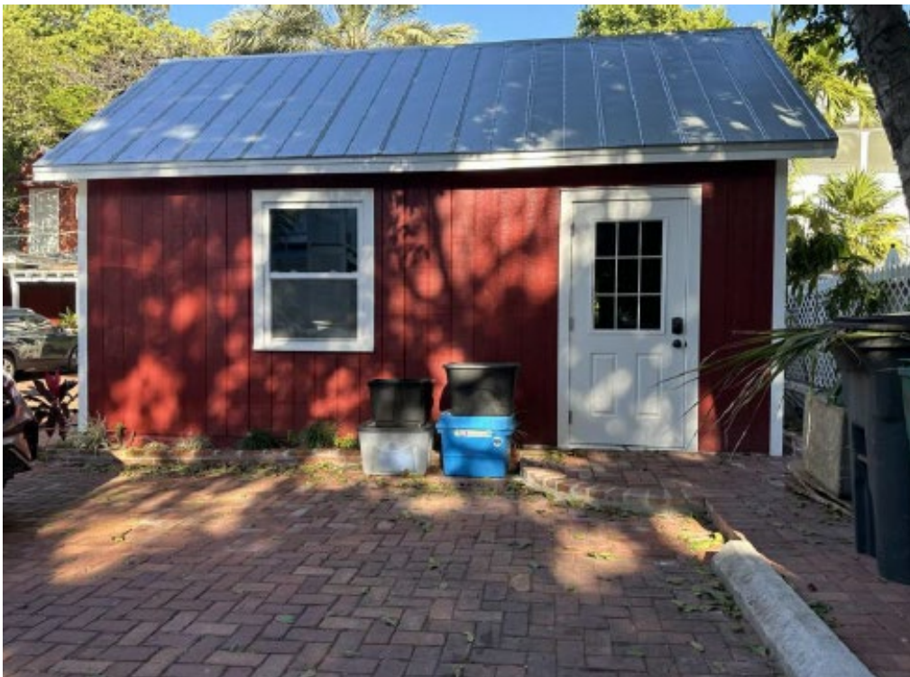
Photo of shed under review (entry elevation).
