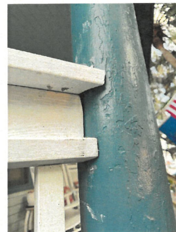
DETAIL - RAILING ATTACHED TO COLUMNS
