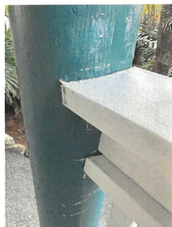
DETAIL - RAILING ATTACHED TO COLUMNS
