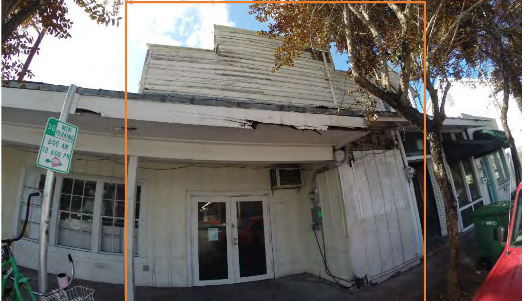
1028 Truman Façade – Stepped Parapet
