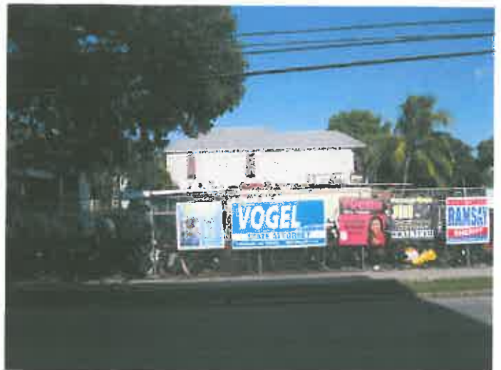
HOUSES BEHIND WELDING SHOP
