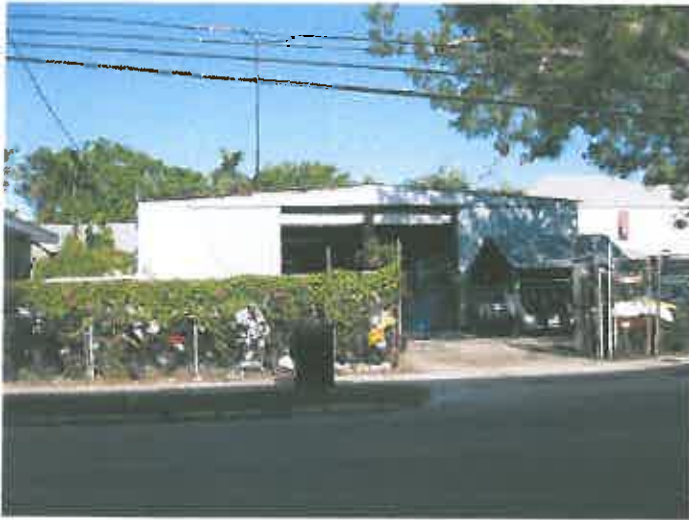
WELDING SHOP FURTHER TO SOUTH
