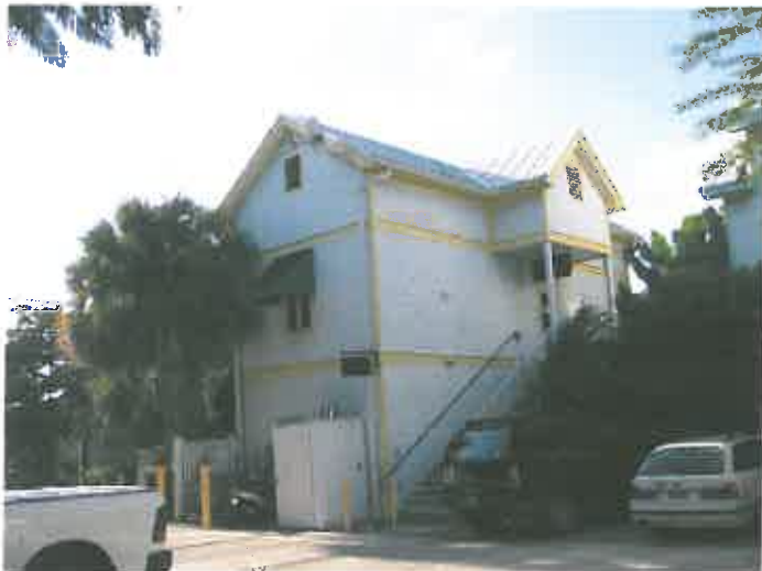
BACK OF BUILDINGS AS SEEN FROM PARKING AREA
