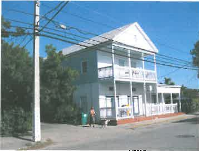
OLD LAUNDRY BUILDING ON CORNER OF VIRGINIA AND SIMONTON
