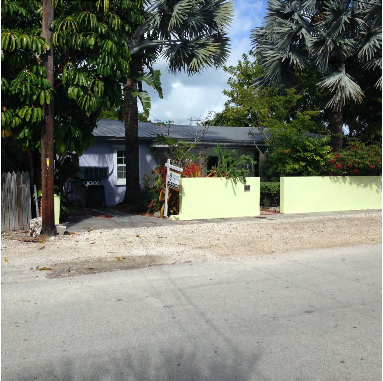
6. Photograph of the adjacent property to the east.
