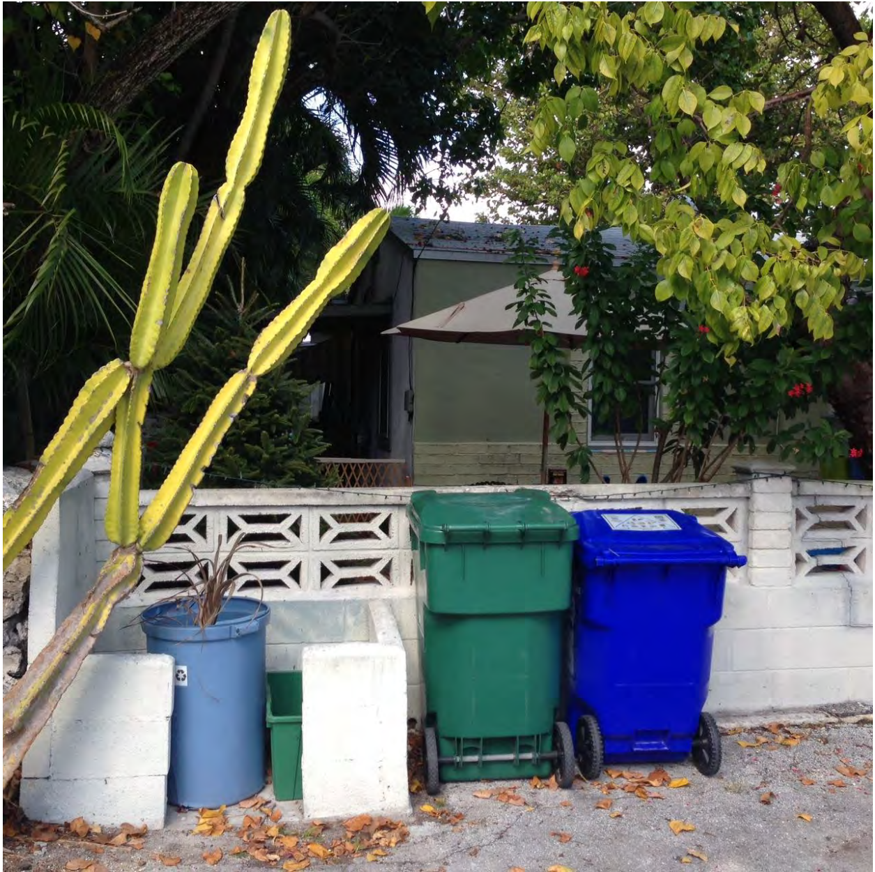
3. Photograph of the west side of the structure.
