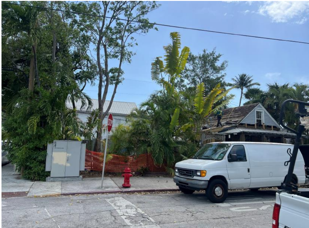
Photo of property under review (currently under renovations).
