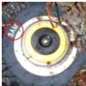
Photo shows “SAM” which stands for seal-a-matic check valve
