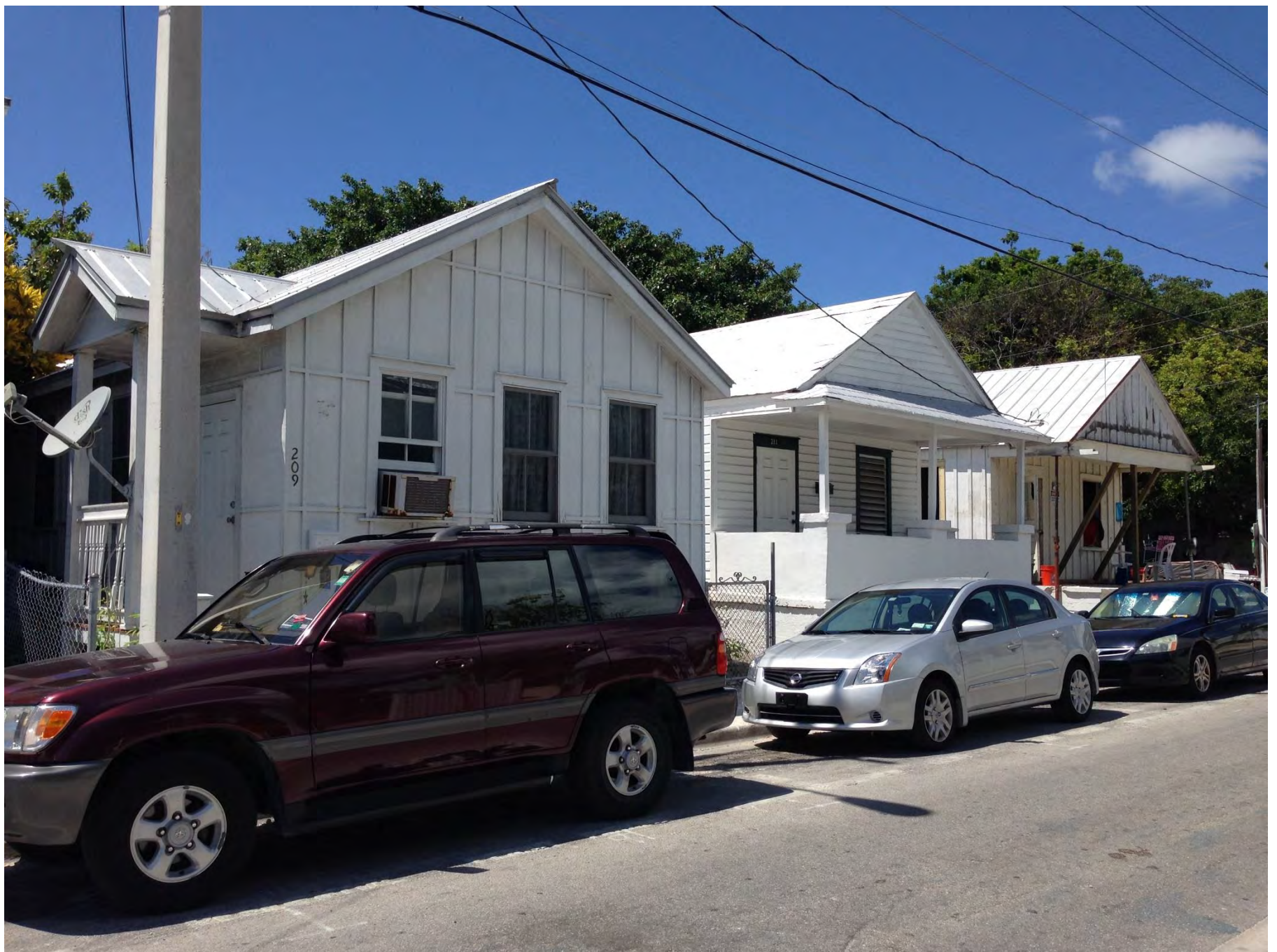
The only small structures in the area. Also across the street on Petronia.
