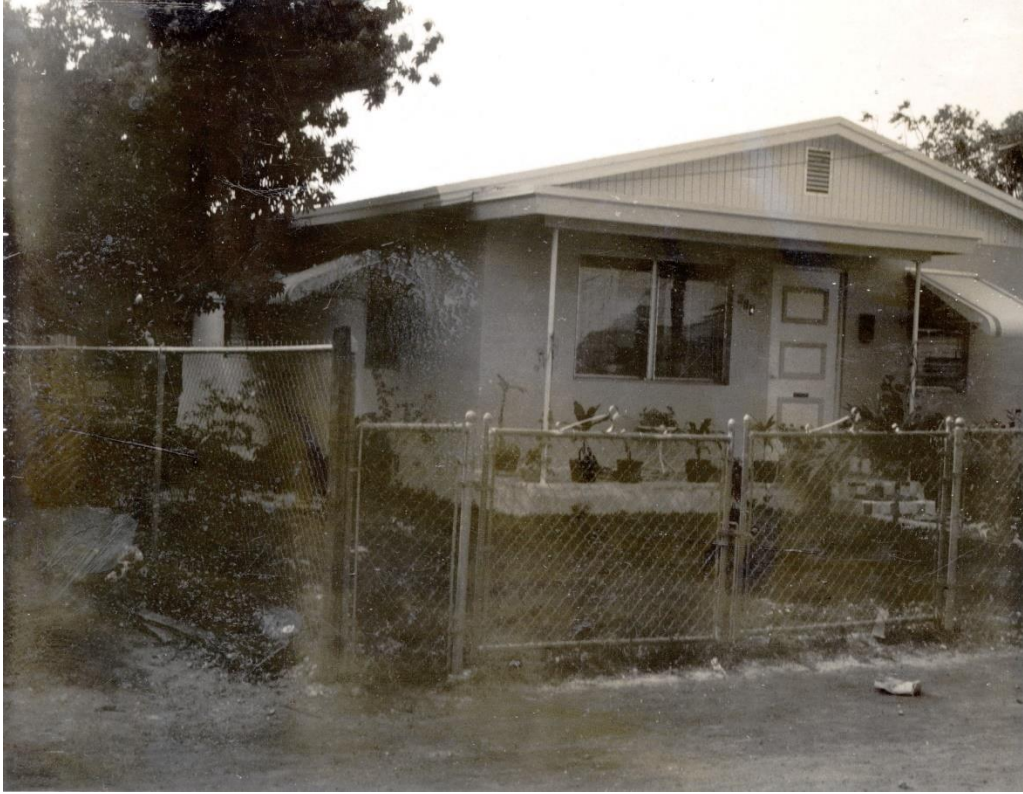
Photo of house under review circa 1965. Monroe County Library.
