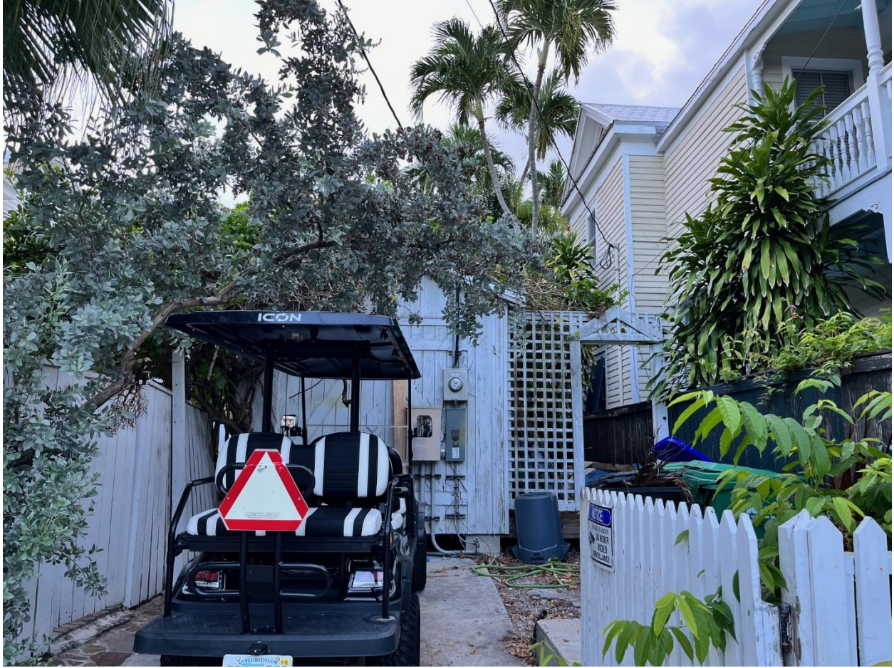
Existing accessory structure view from Grinnell Street.
