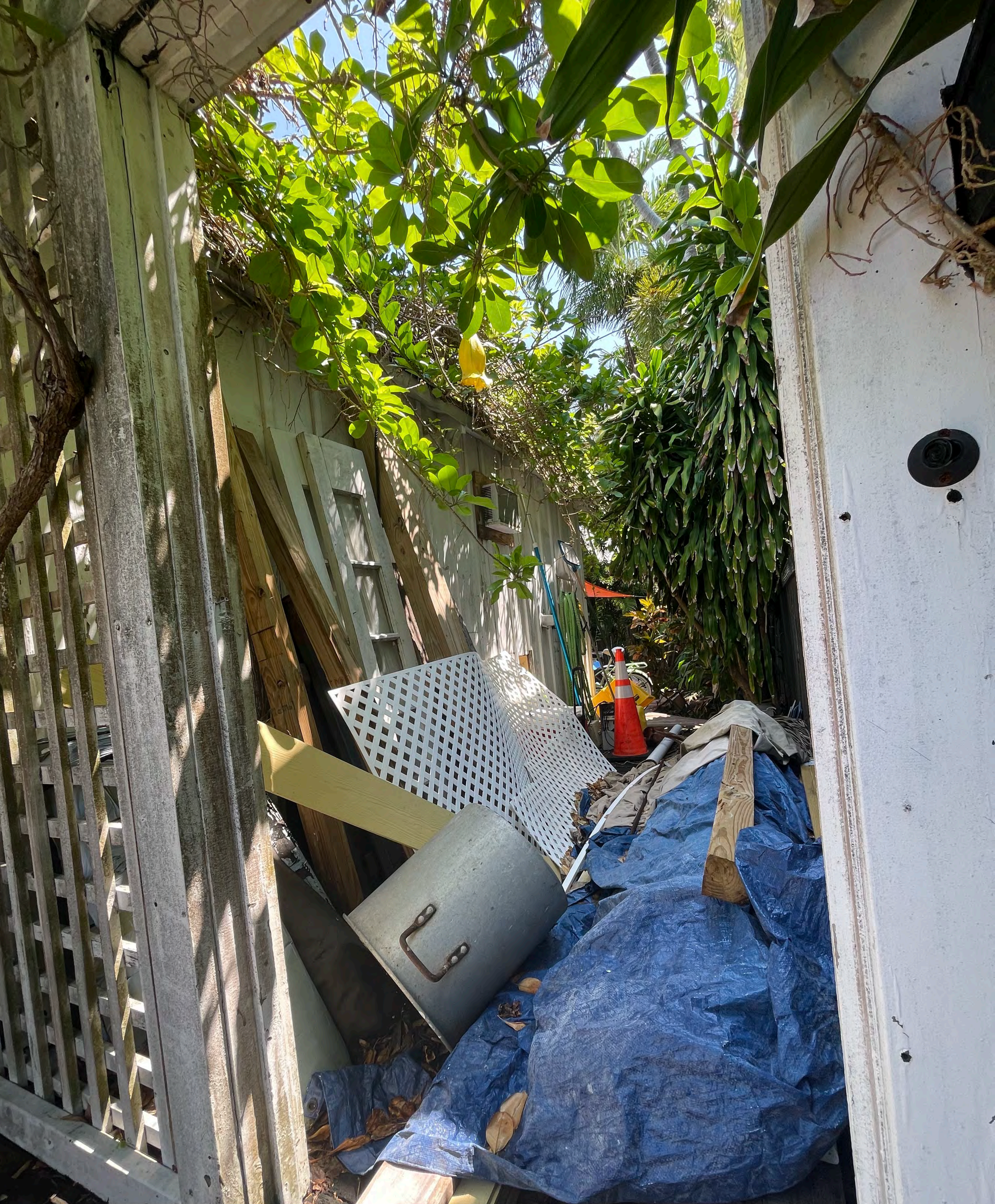
1002 Fleming Street existing accessory structure view along south side
