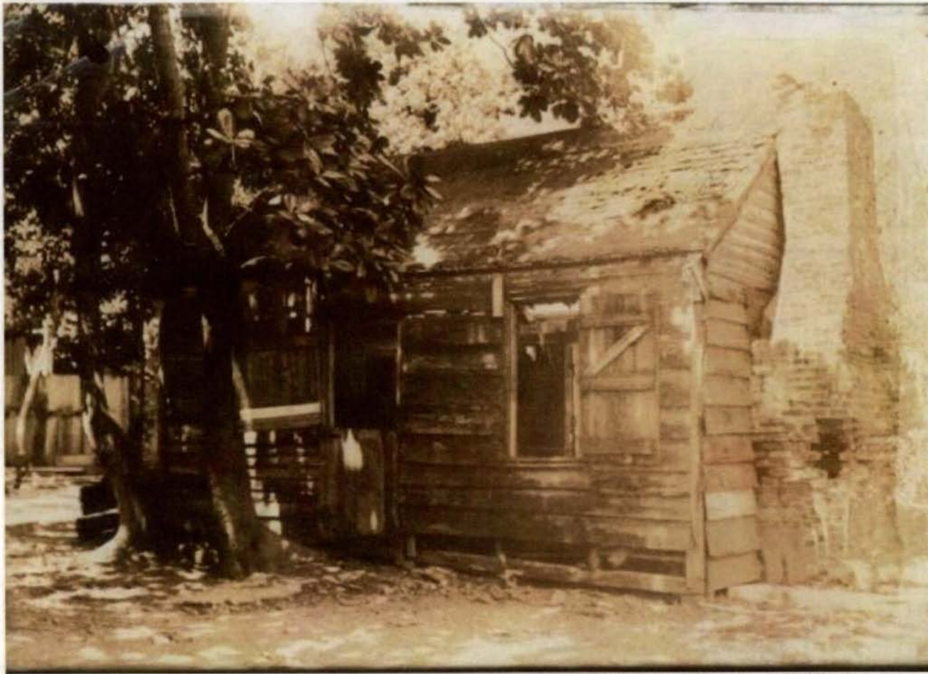
1916 photo of Key West kitchen
