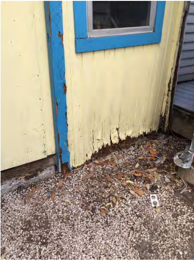
Shed to be demoed
