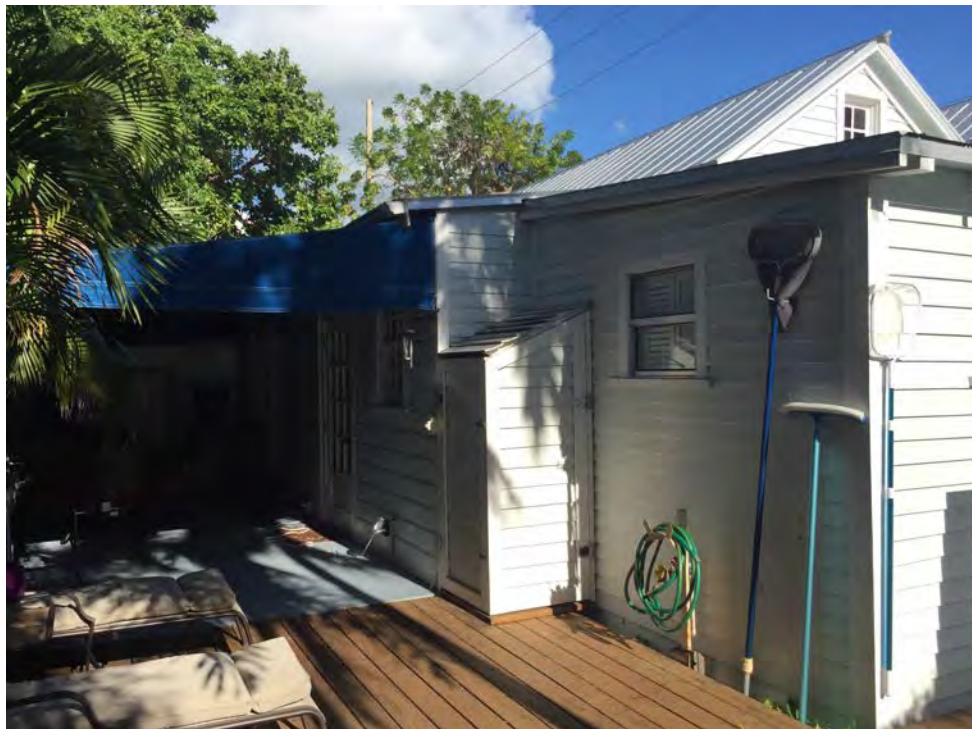
Rear Yard – shed roof (parallel to gable roofs) to be demoed
