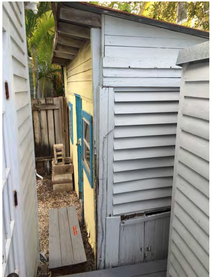
East Side Yard – shed to be demoed
