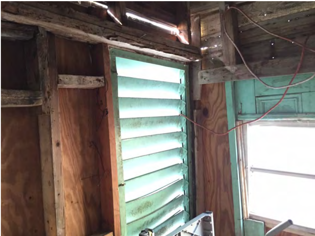
Interior of shed to be demoed
