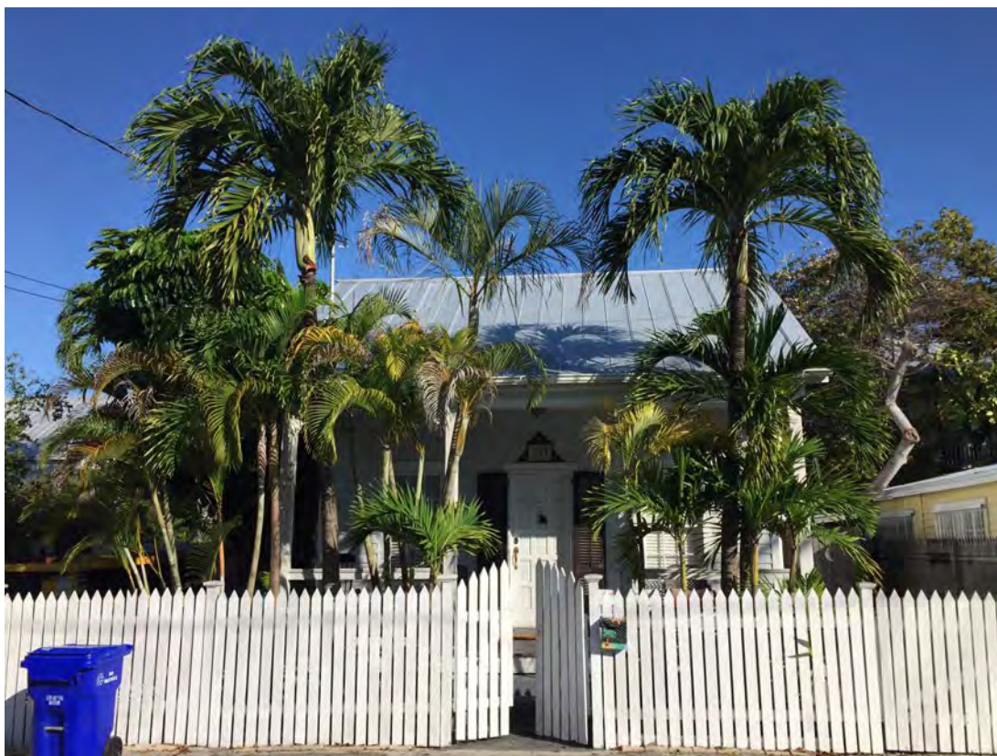
Front View / South Elevation
