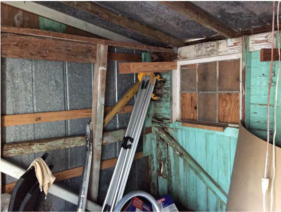
Interior of shed to be demoed
