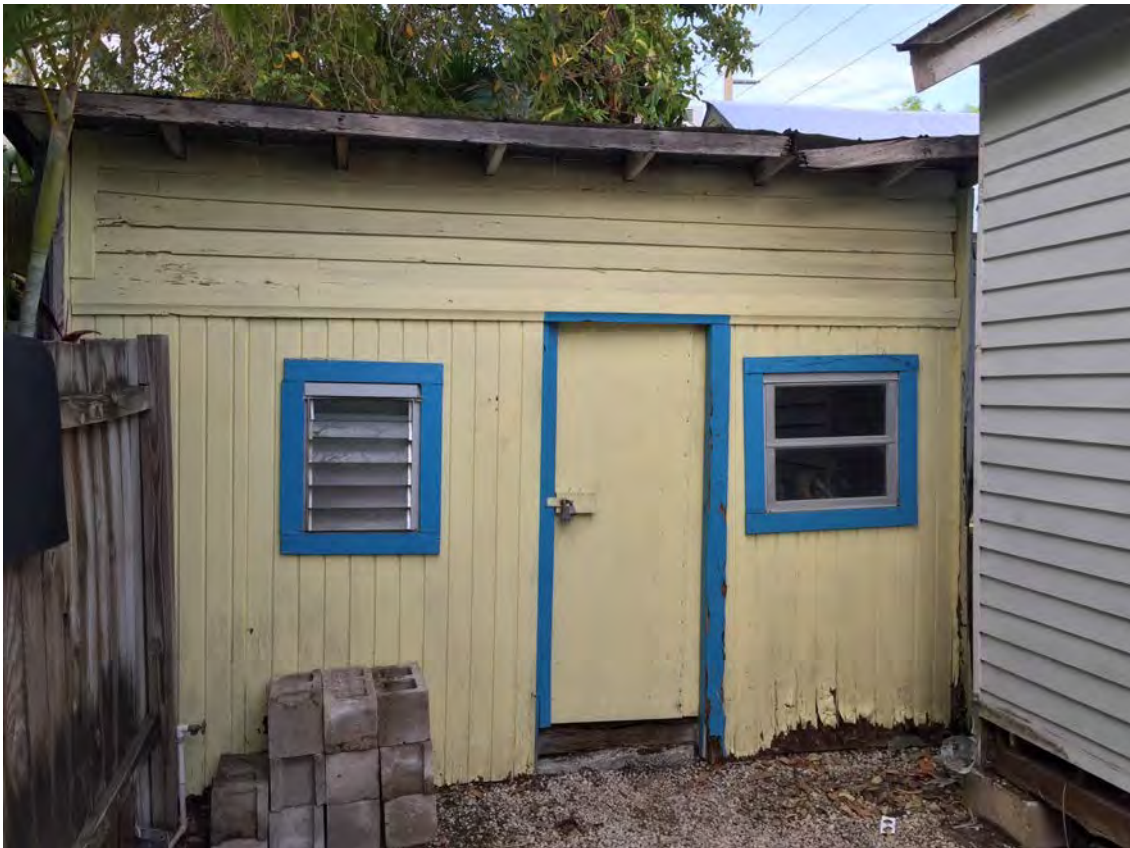
Shed to be demoed
