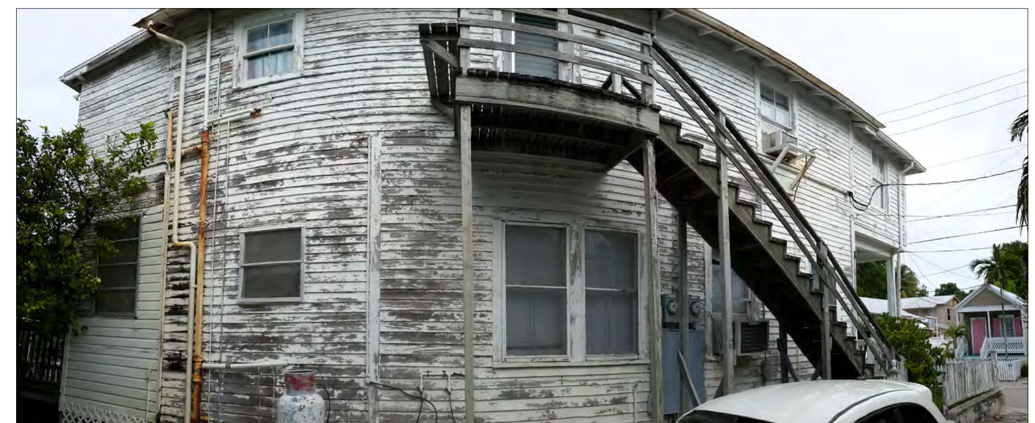
LOOKING NORTHEAST (SIDE)
