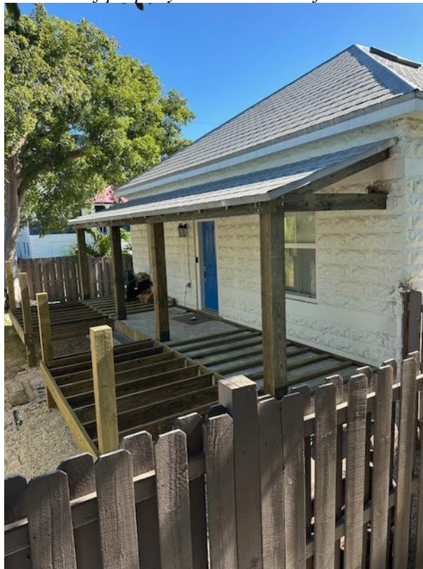
Photo of property under review during construction.
