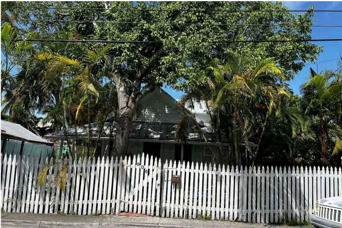
Current photo of house under review.
