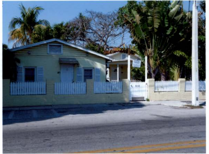
Fence to right of entrance gate must be replaced
