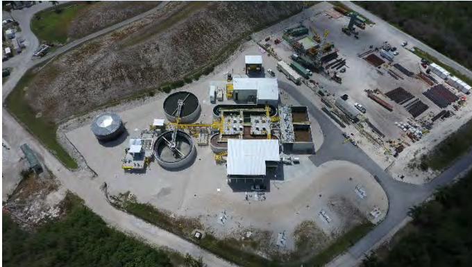
Complete Cudjoe Regional AWRF with Deep Well construction underway
