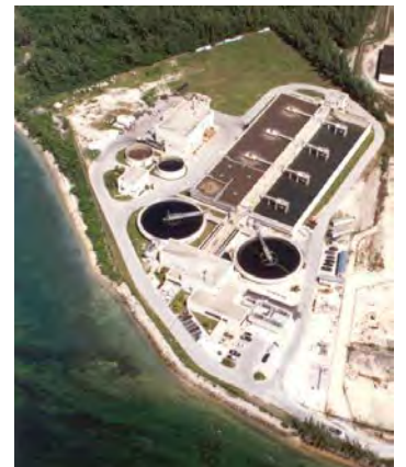
Improvements to pump station and utilization of abandoned piping have allowed the City to increase flows to the Richard A. Heyman EPF.
