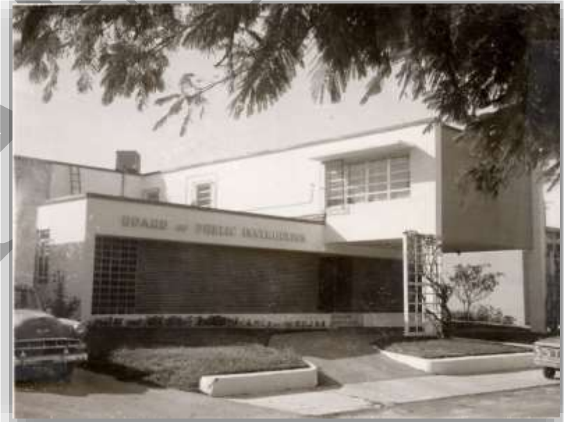
500 Whitehead Street- Monroe County Library ca. 1965
