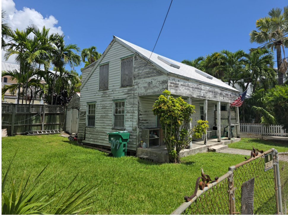
NORTH SIDE OF RESIDENCE
