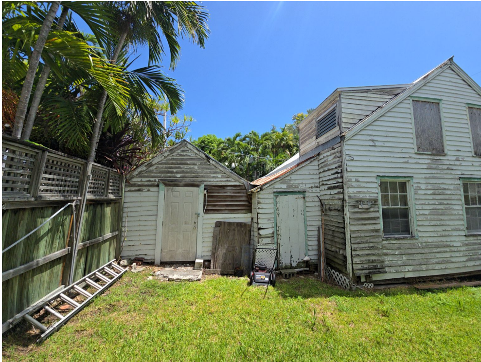
NORTH SIDE OF RESIDENCE
