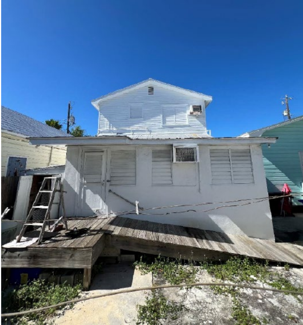
Photo of rear of Property Under Review.
