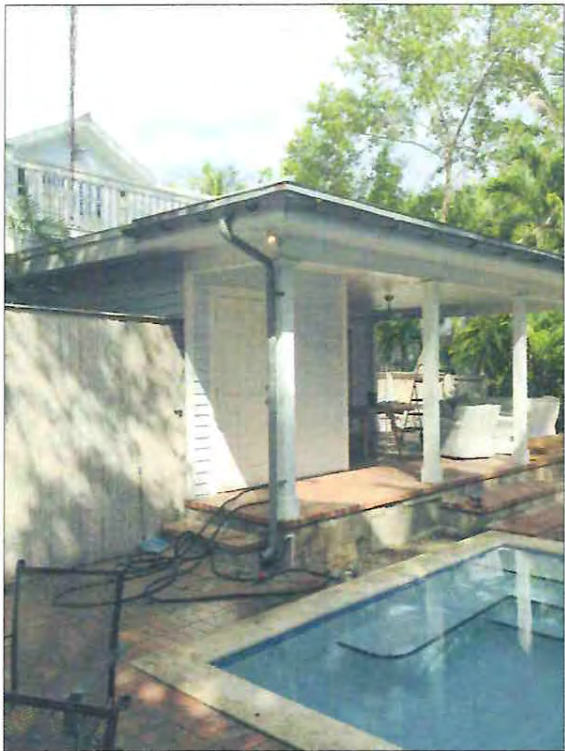
FIGURE 3 VIEW FROM REAR OF HOUSE
