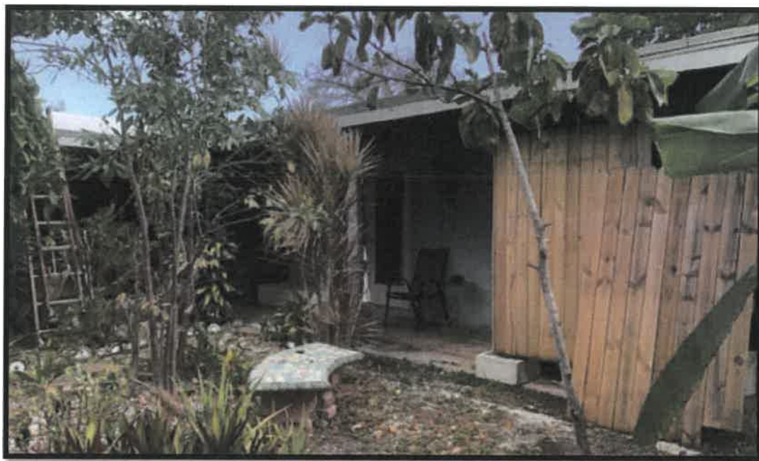
Lockout Unit attached to unit #9 - exterior
