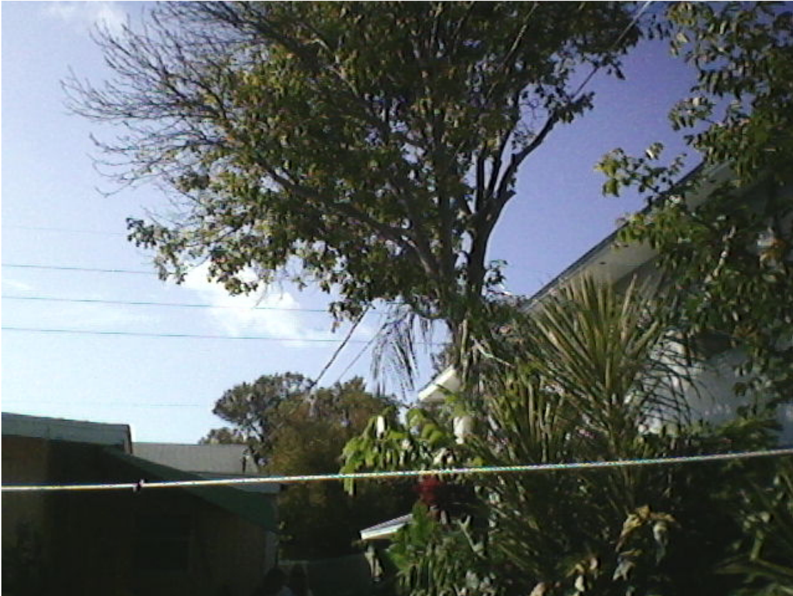
Picture of tree showing tip die back and proximity to wall
