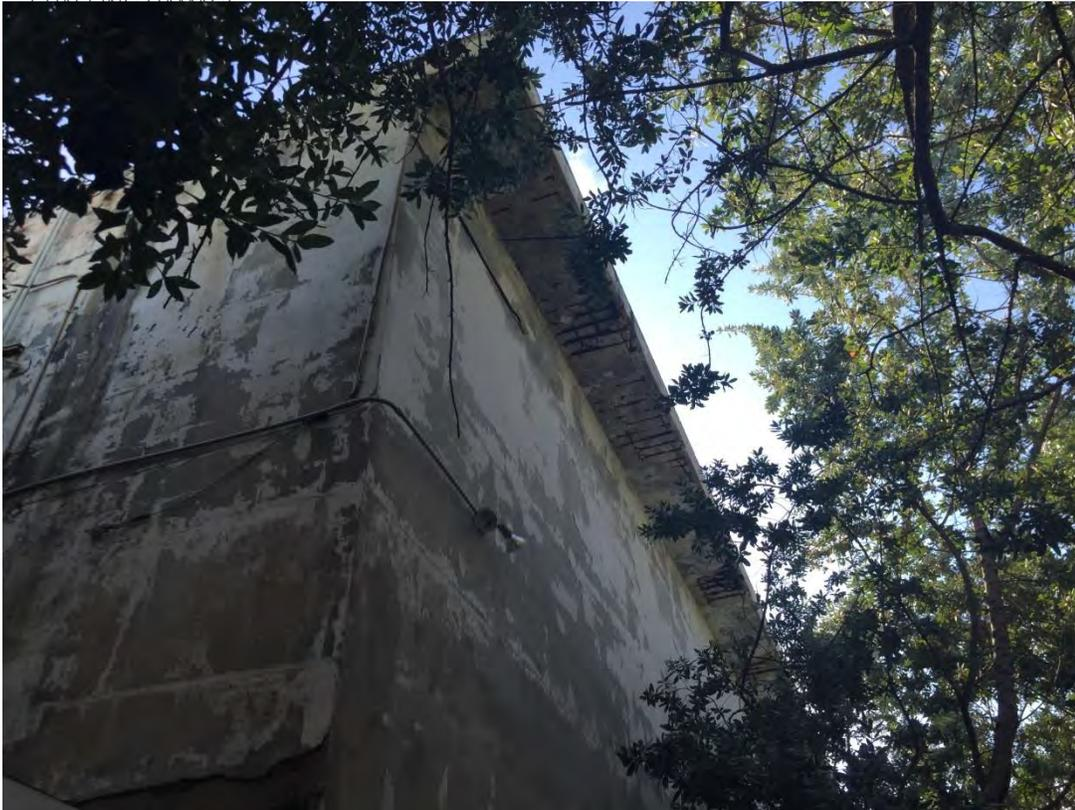
REAR FAÇADE - EXISTING ROOF CONDITION WITH SPALLING DAMAGE
