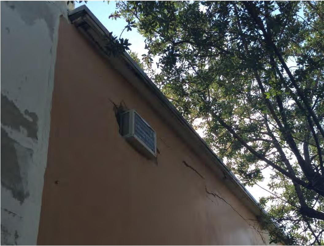
SPALLING DAMAGE AT EXISTING REAR FACADE
