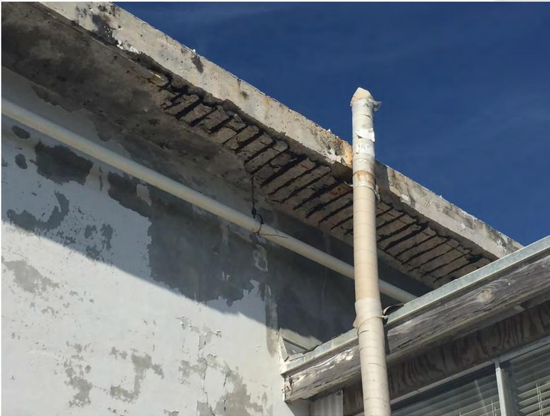
FRONT FAÇADE - EXISTING ROOF CONDITION WITH SPALLING DAMAGE
