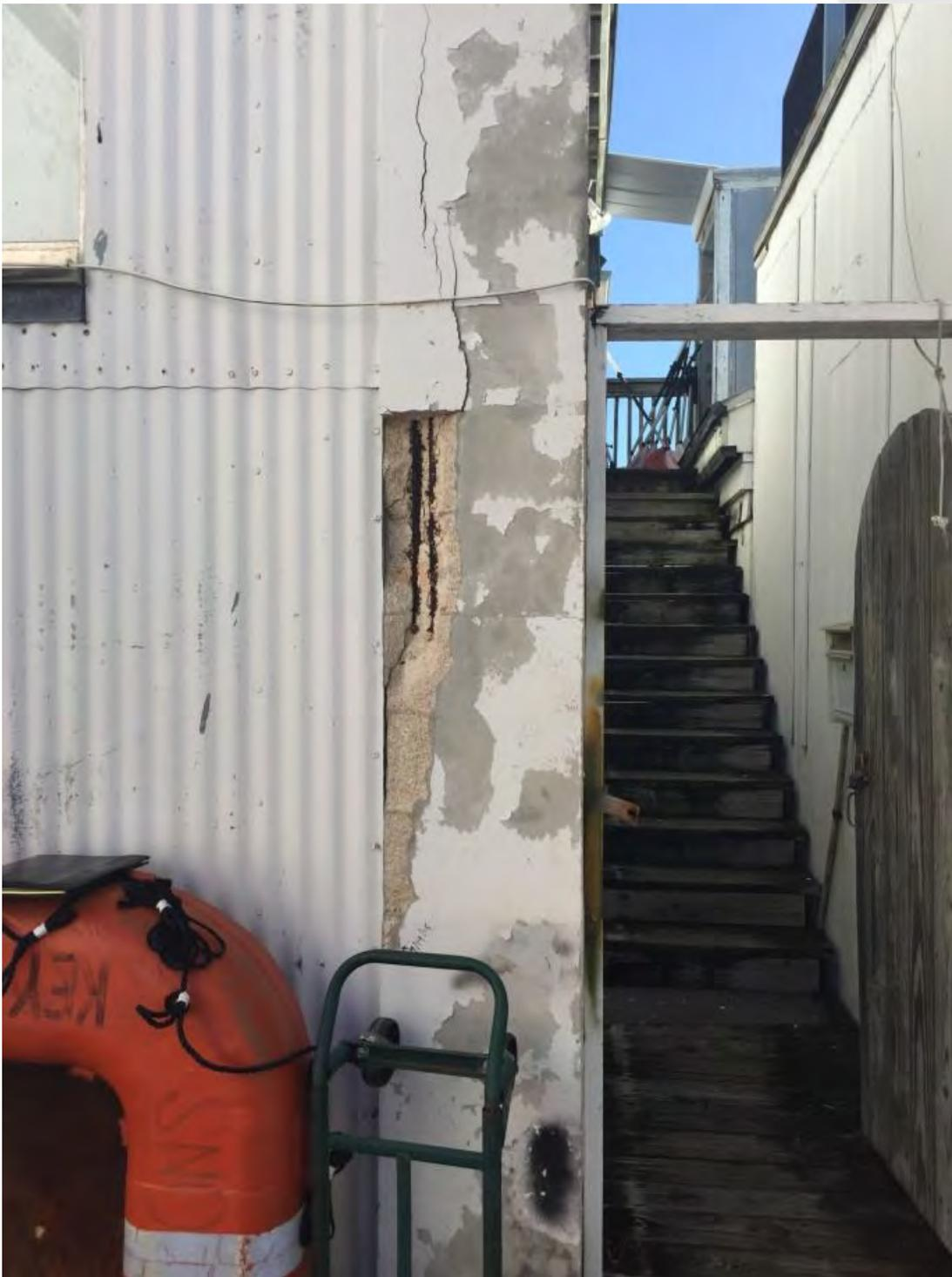
SPALLING DAMAGE AT EXISTING CONCRETE COLUMN
