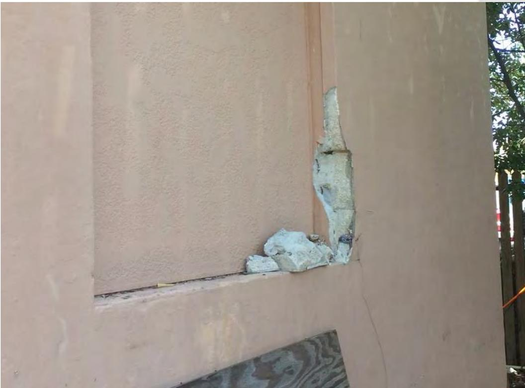
SPALLING DAMAGE AT EXISTING REAR FACADE
