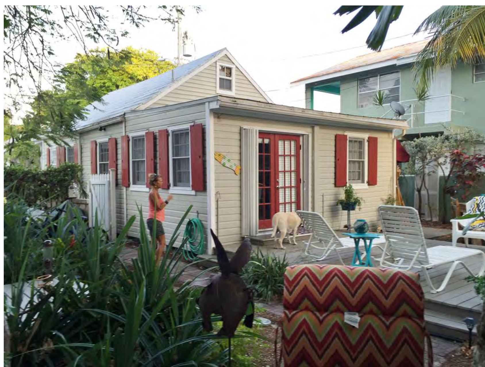
BACK ELEVATION, PHOTO 3
