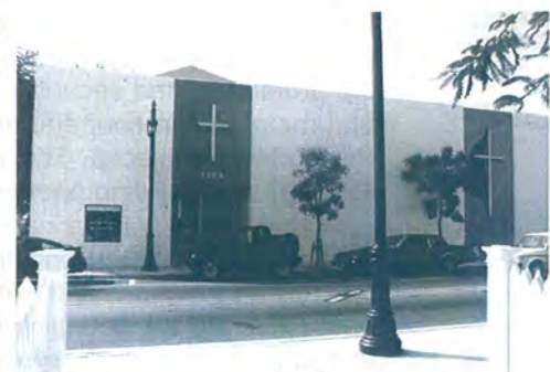
Same view prior to removing 1960's addition th obscured the Sanctuary. Sanctuary windows were intact behind the addition, but the front porch required reconstruction. Note the Sanctuary roof above the 1960's addition.
