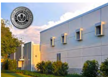
Seminole Public Works Operations
