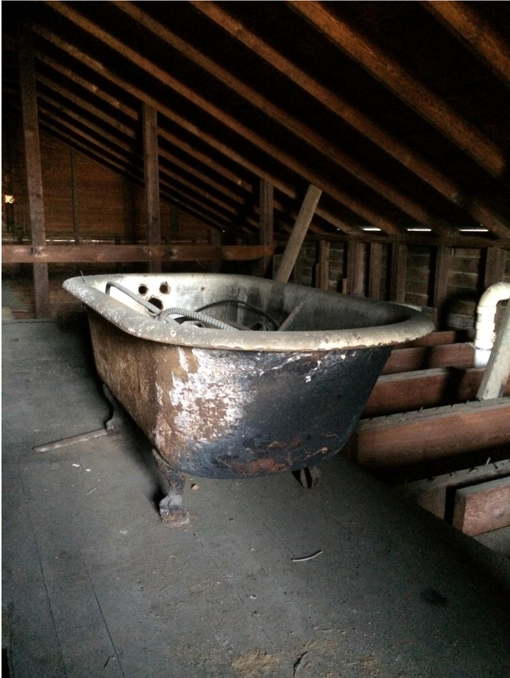
Photo: Existing Conditions; Original Clawfoot Bathtub
