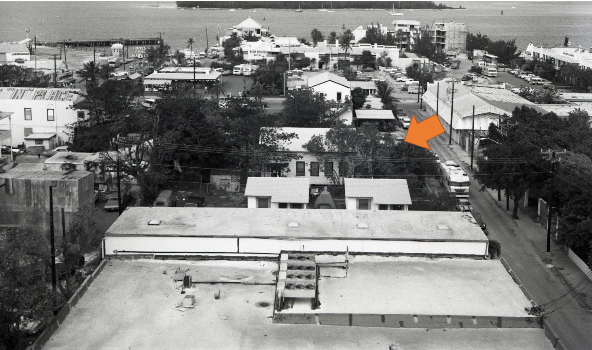
1970s Photograph from Old City Hall. Monroe County Public Library.
