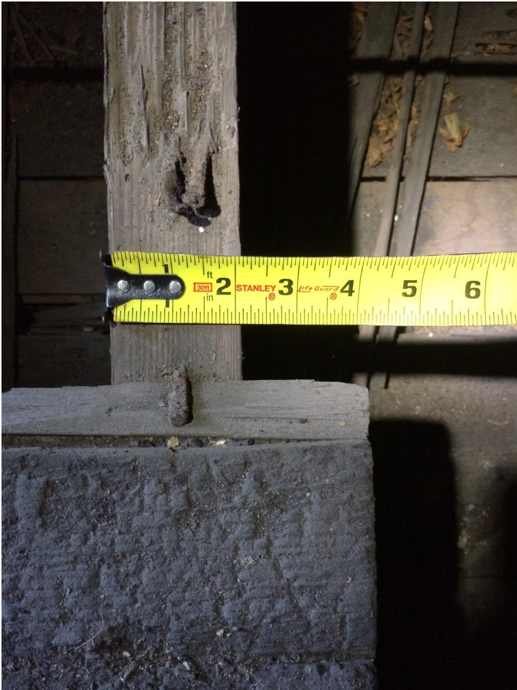
Photo: Existing Conditions; Original 2" Lumber
