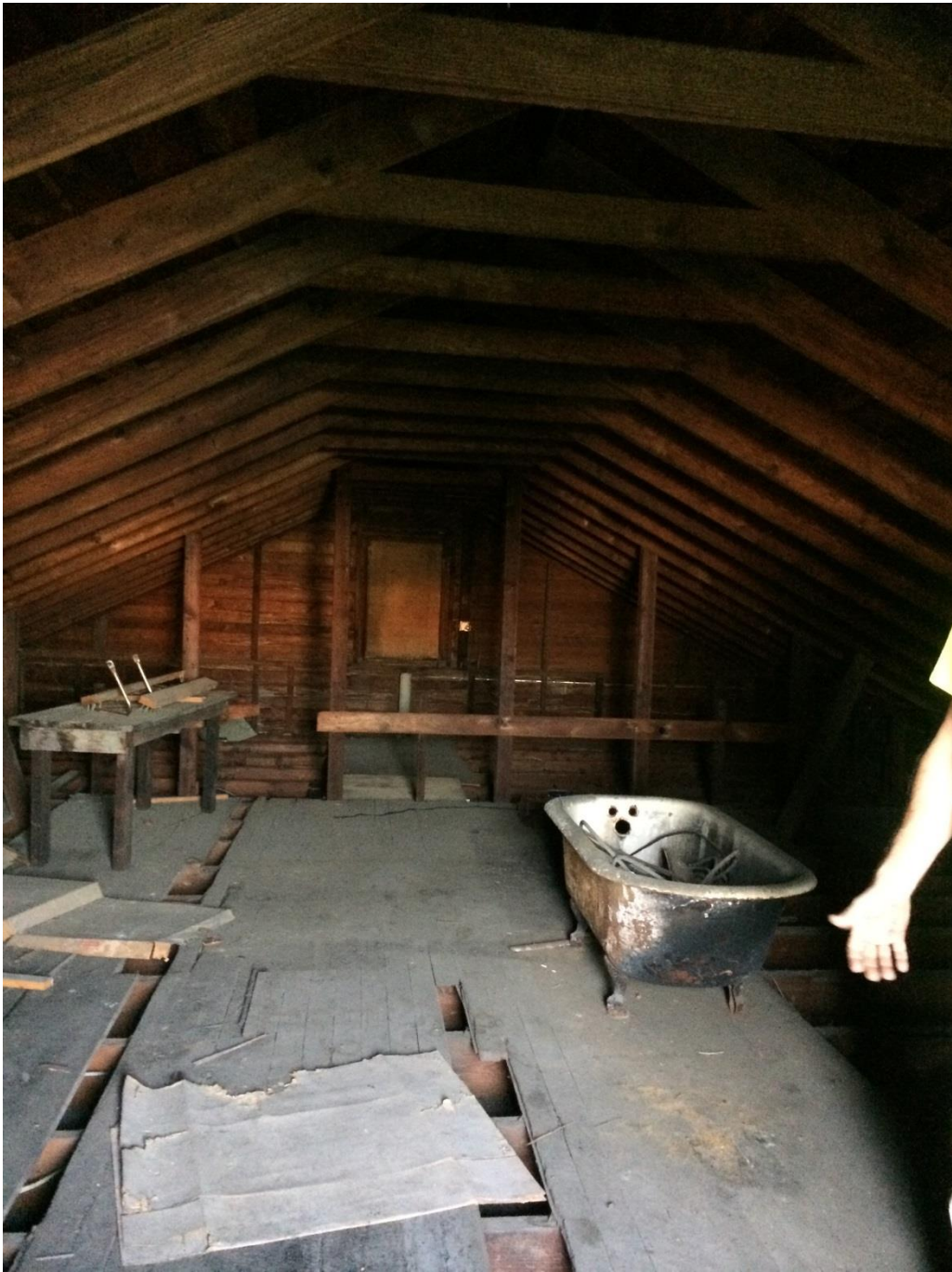
Photo: Existing Conditions; Attic Facing Bagatelle
