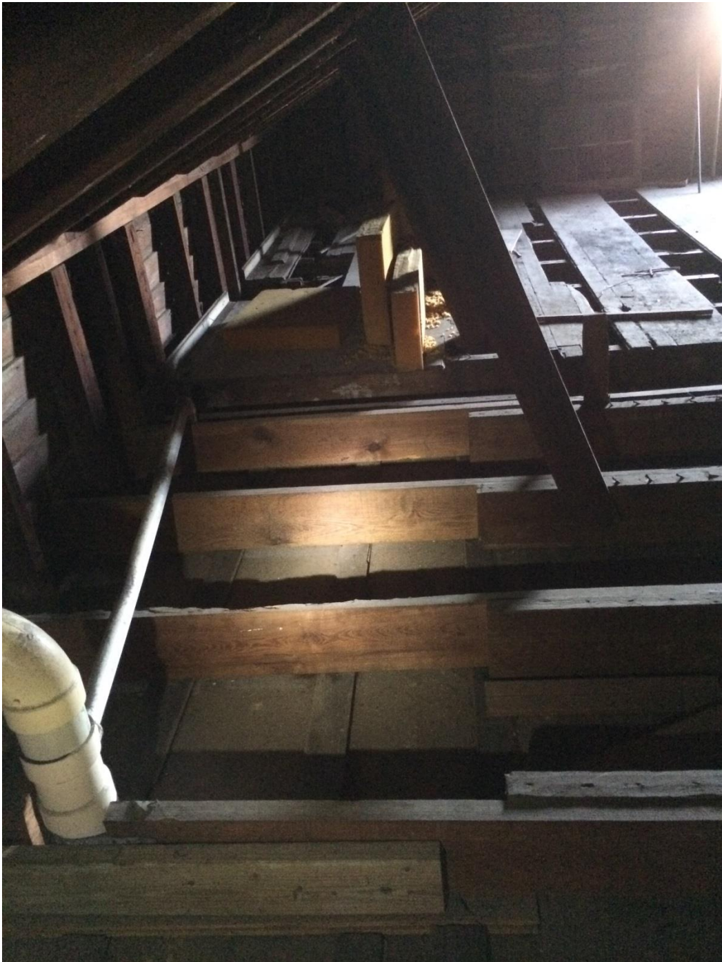
Photo: Existing Conditions; Original Stair Opening
