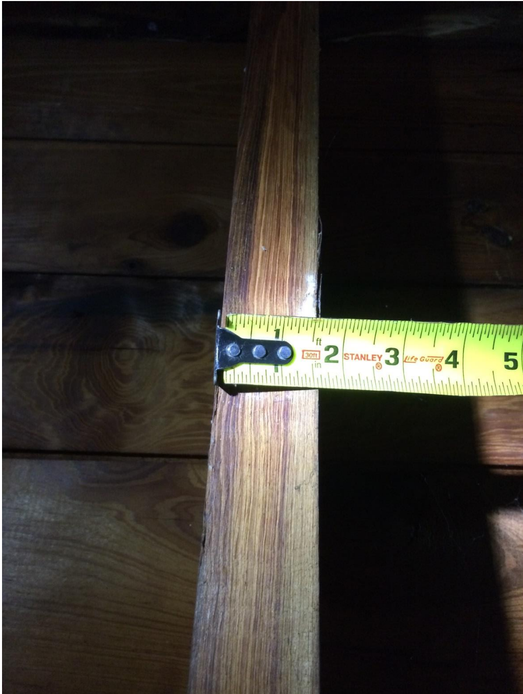
Photo: Existing Conditions; New 1-1/2" Nominal Lumber
