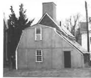
Temporary stabilization or "mothballing" with materials, such as plywood and building paper, can protect the roof of a project until it can be properly repaired or replaced. Photo: NPS files.
