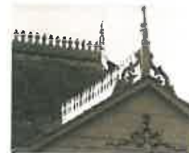
Decorative roofing feature. Photo: HABS Collection, NPS.
