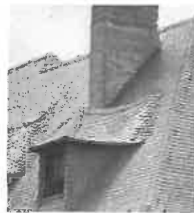
Because of the roof's visibility, the slate detailing around the dormers is important to the character of this structure. Photo: NPS files.
