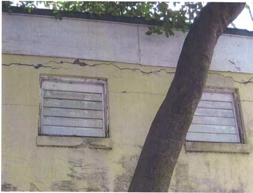
Detail photo of 2 nd floor spalling tie beam at north façade. Contractor to repair spalling at tie beams and columns and patch stucco. See structural details and specifications.
